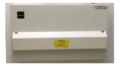
If for any reason the unit requires isolating, this is achieved by carefully lifting up the front cover, which will expose the circuit breakers and switching the main incoming isolator (Red in colour and marked MAIN SWITCH) to the off position. Should one of the circuits trip, lifting the front cover will show any circuits that have tripped and they can be reset, should the circuit persistently trip please contact the Residents Team as soon as possible.
