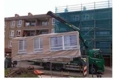
External insulation and prefabricated building elements
