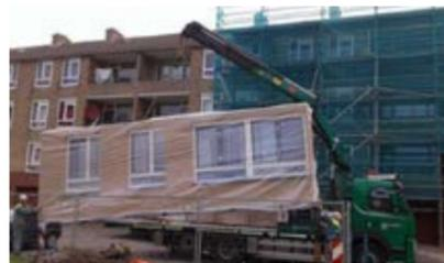
External insulation and prefabricated building elements
