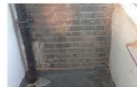
One bed flats have small balconies
