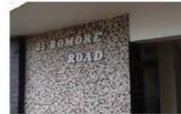
Original signage is in good condition
