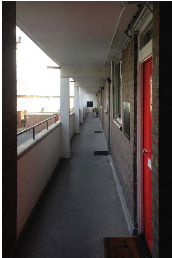
Existing deckway condition
