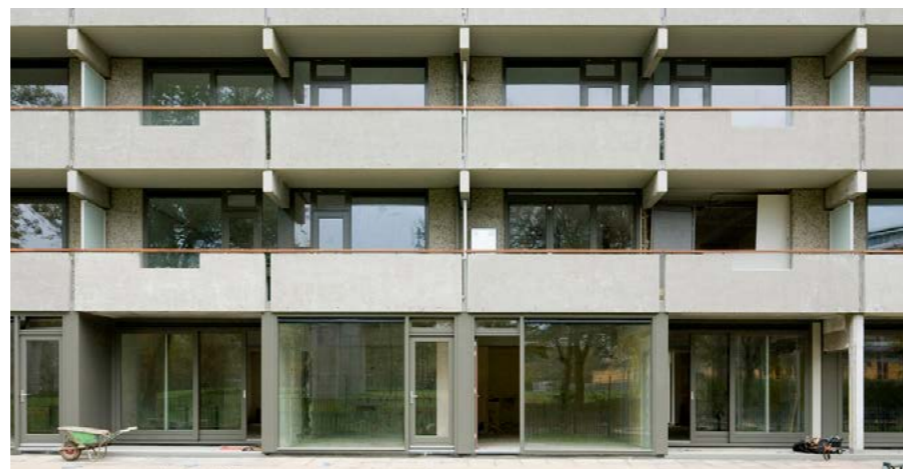
Example of new windows in an existing block. (Image: NL Architects)
