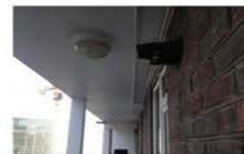
Homes have individual boilers
