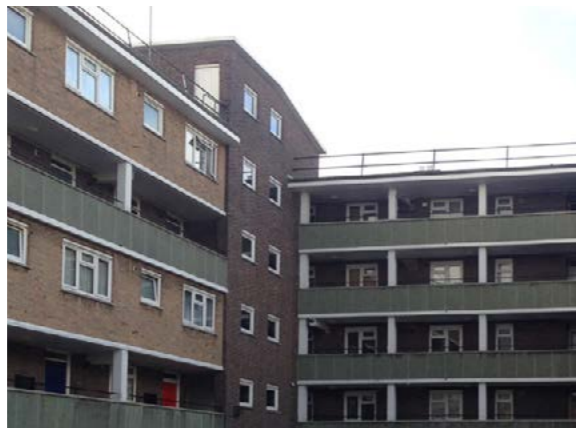
Existing deckway condition
