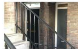
Doorways are recessed
