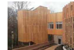
Example of timber stair
