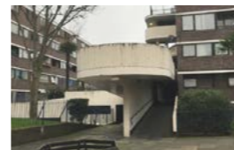
The ramps are barrier to movement around the estate.
