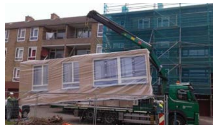
External insulation and prefabricated building elements
