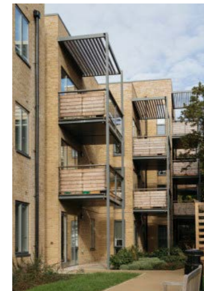
Example of a balconies with a cover for solar shading
