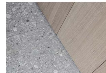
Terazzo floor & timber doors
