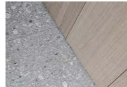
Terrazzo floor & timber doors
