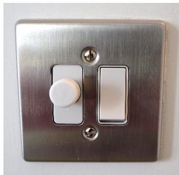
Kitchen Dimmer Switch
