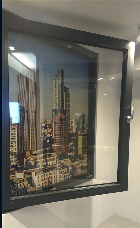
Bidix: Tusaalayaasha daaqada lamid ah ee janjeedhka ah iyo leexda ee tijaabada lagu xidhay MidigL. Tusaalaha fireemka almuuniyeemka ah
