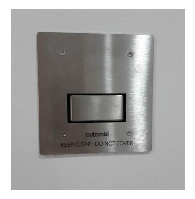
The refurbishment of this flat included the instalment of a new fire detection and suppression system, called **The Plumis Automist Smartscan Hydra**.
