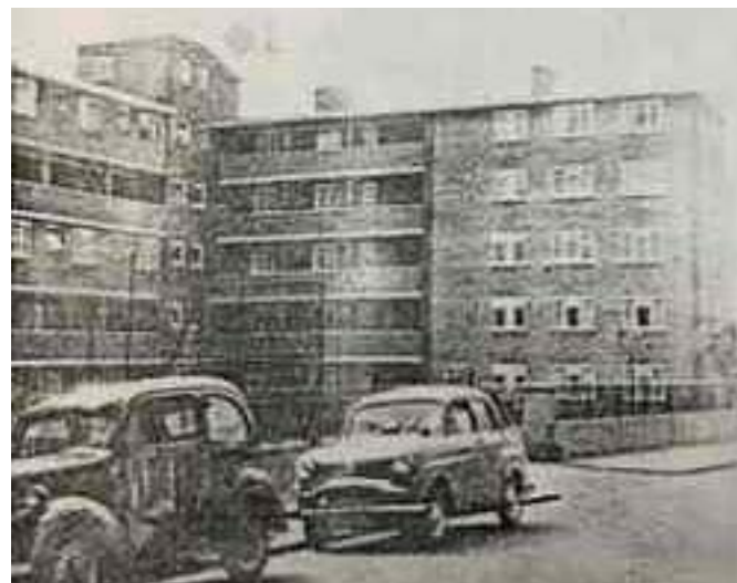
Lancaster West Estate Refurbishment
