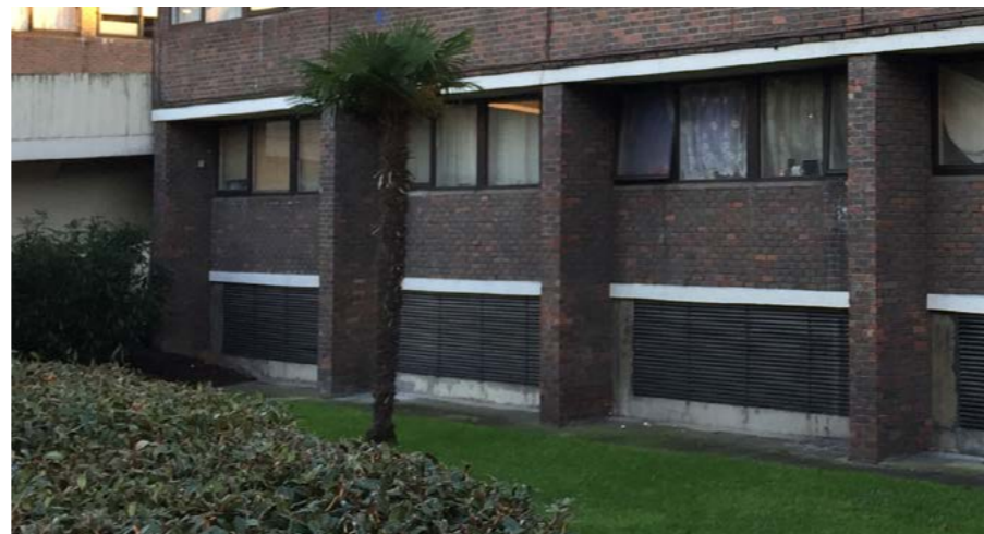
Lack of overlooking at ground floor level
