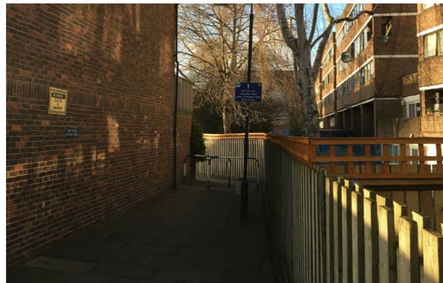
Safety concerns along pedestrian routes
