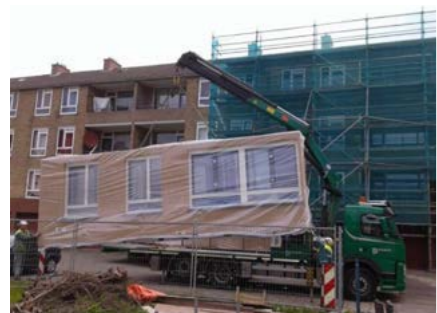
External insulation and prefabricated building elements
