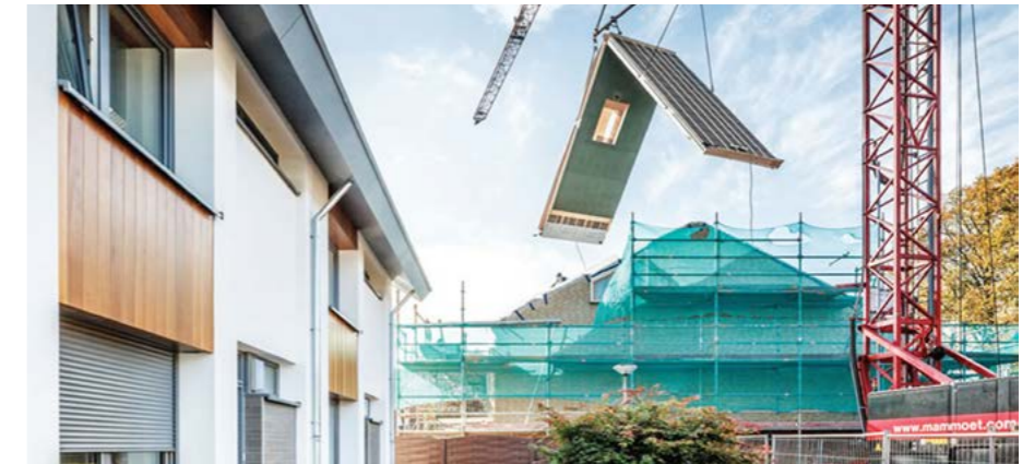
Dutch example of new insulated roof in one-week complete refurbishment
