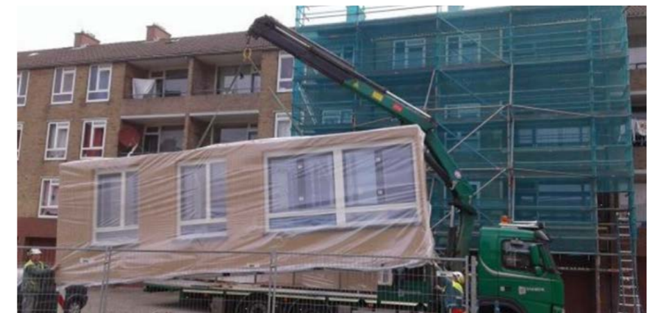
Prefabricated modules installed from outside to minimise resident disturbance
