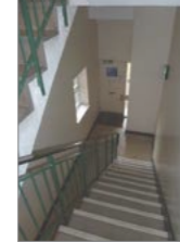
Block 2 communal stairwell
