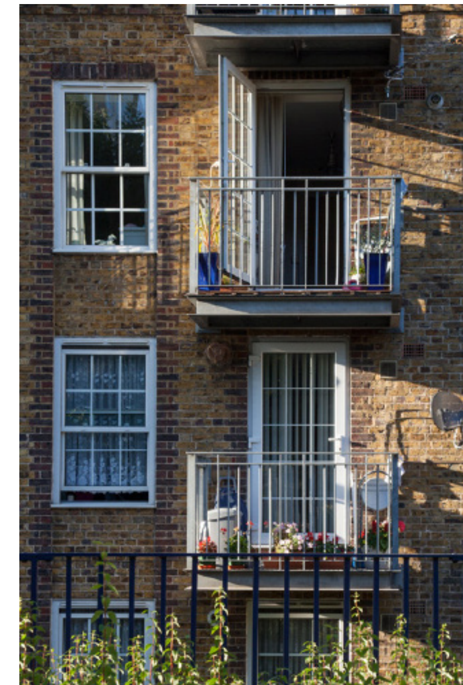
Example of a "bolt-on" balcony
