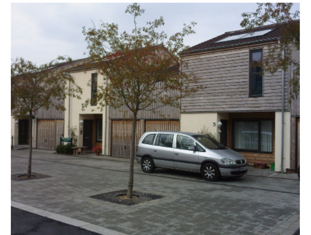
Shared surface with level access to homes
