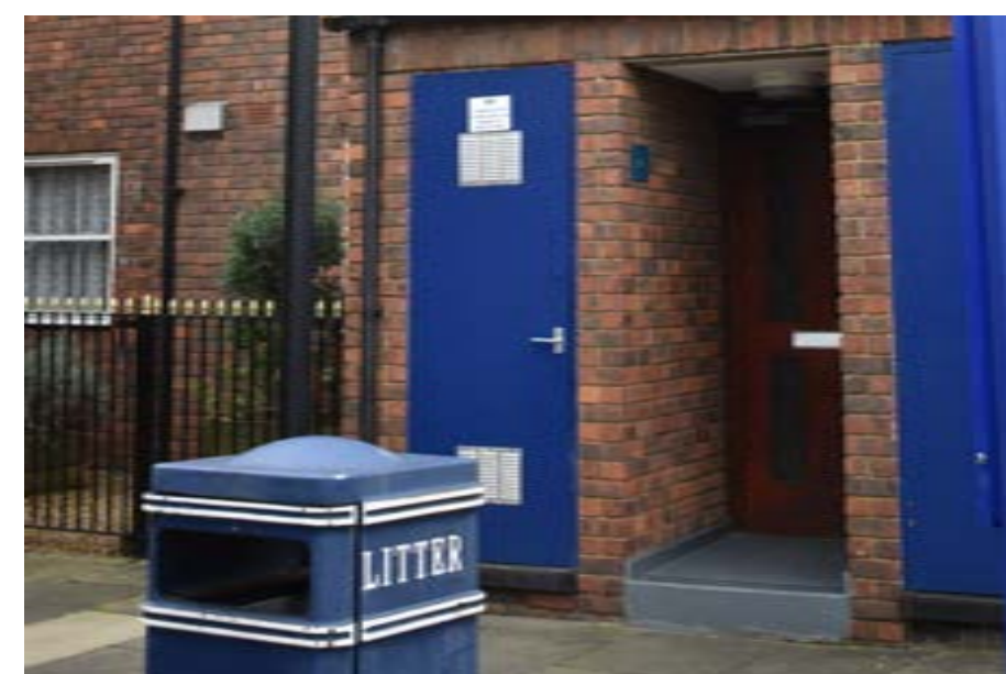
Stepped entrances to homes
