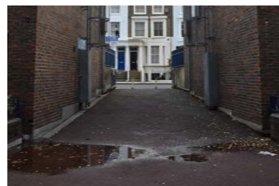
Walkway constantly floods
