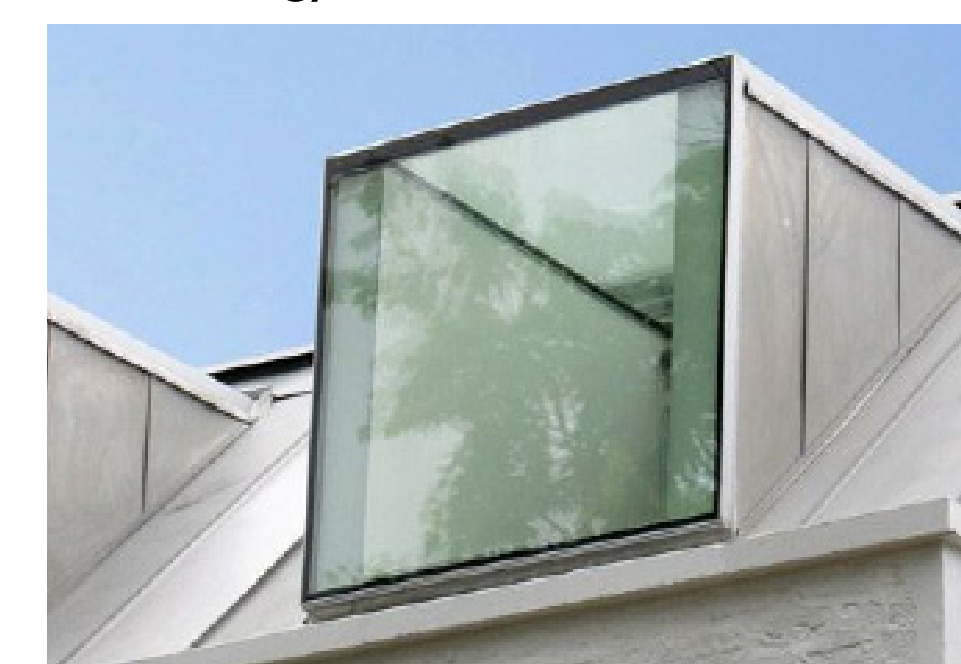
Dormer window upgrade: more usable space
