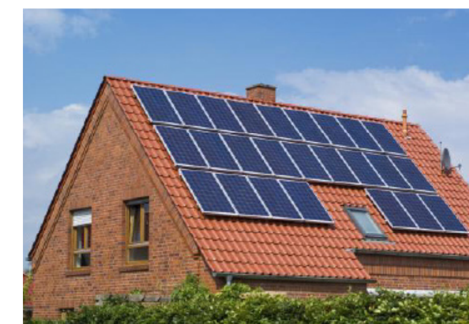
3 PV solar panels on roof: reduce energy bills
