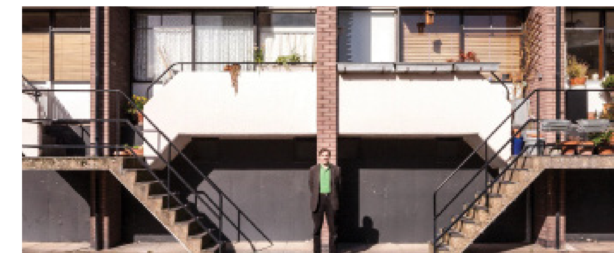
Example of well designed steps to link lower flats to courtyard spaces
