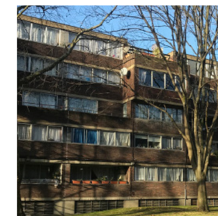
Existing separation of flats from the courtyard
