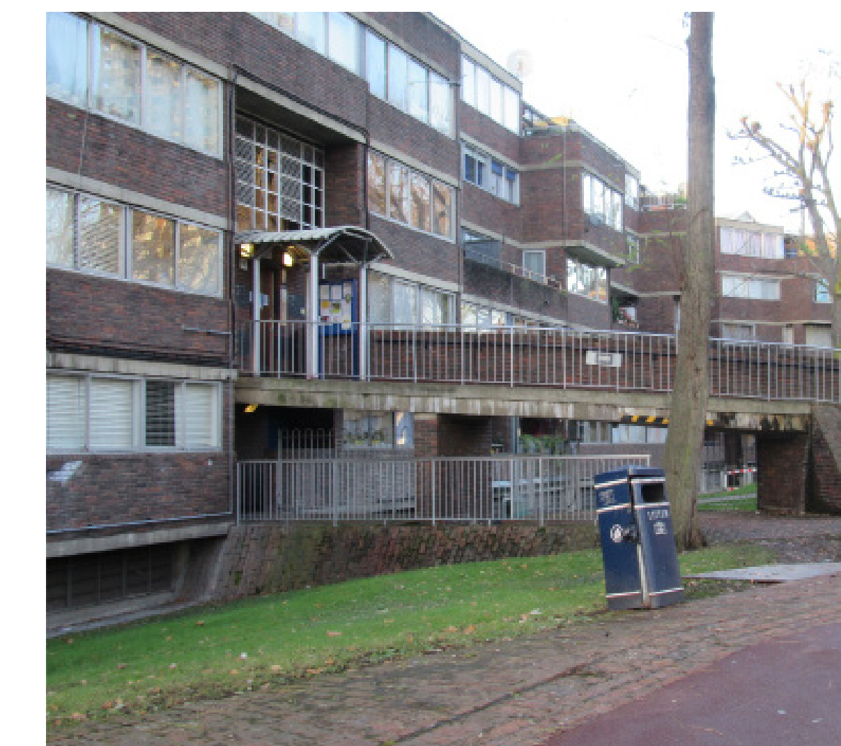
Existing ramped entrances within courtyards
