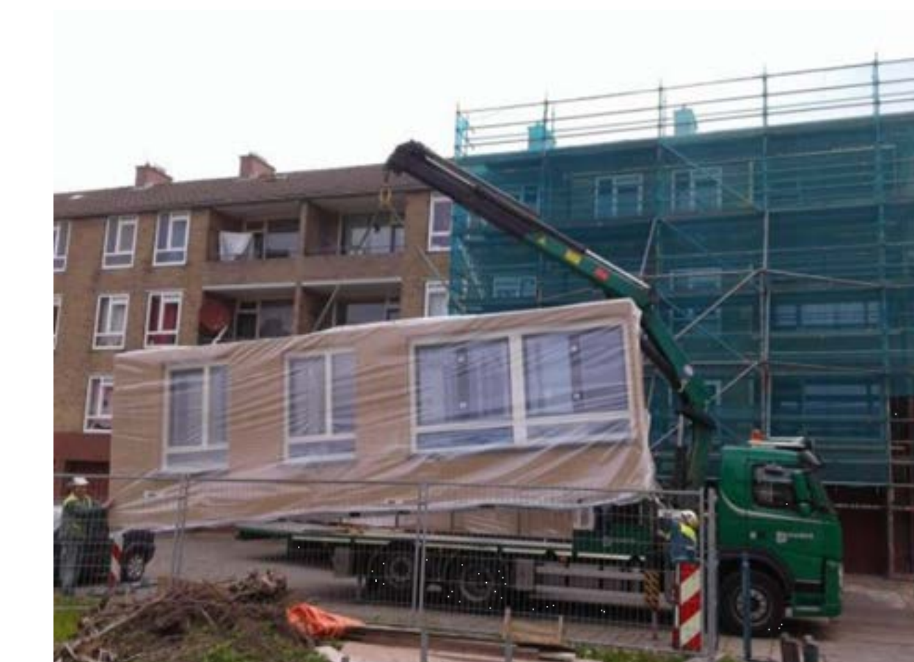
External insulation and prefabricated building elements
