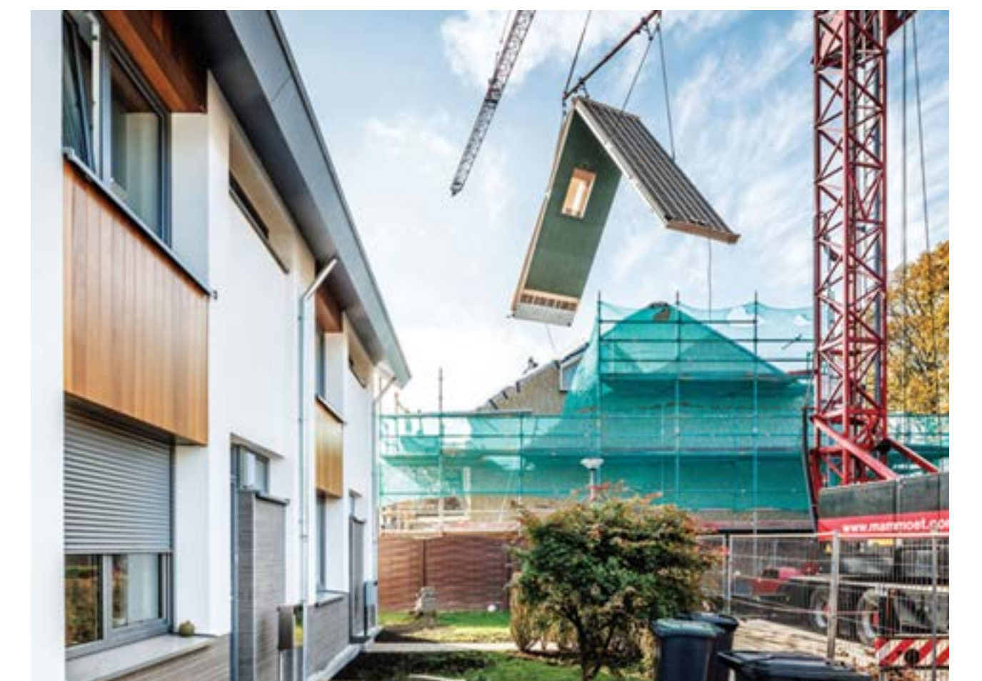
Prefabricated elements to reduce disruption and improve performance
