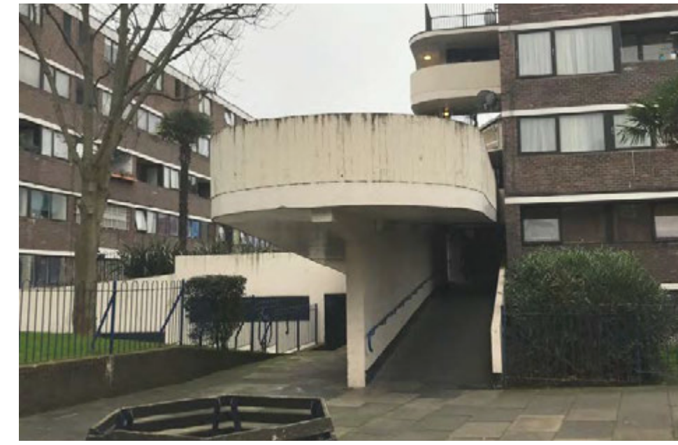
The ramps are barrier to movement around the estate.
