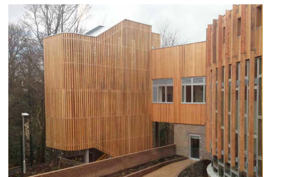
Example of timber stair
