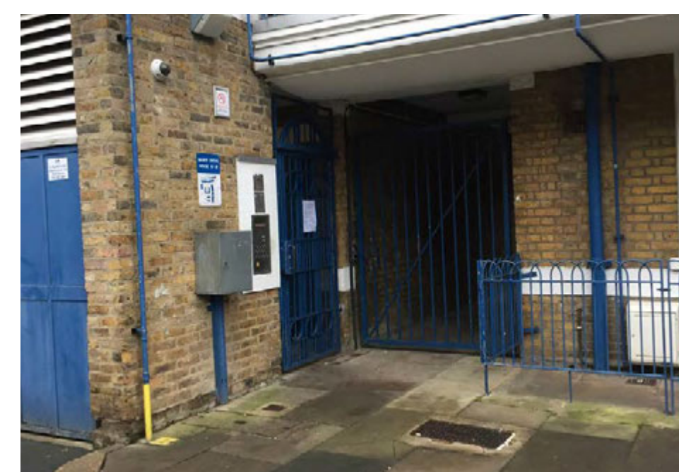
Entrances areas not clearly identified
