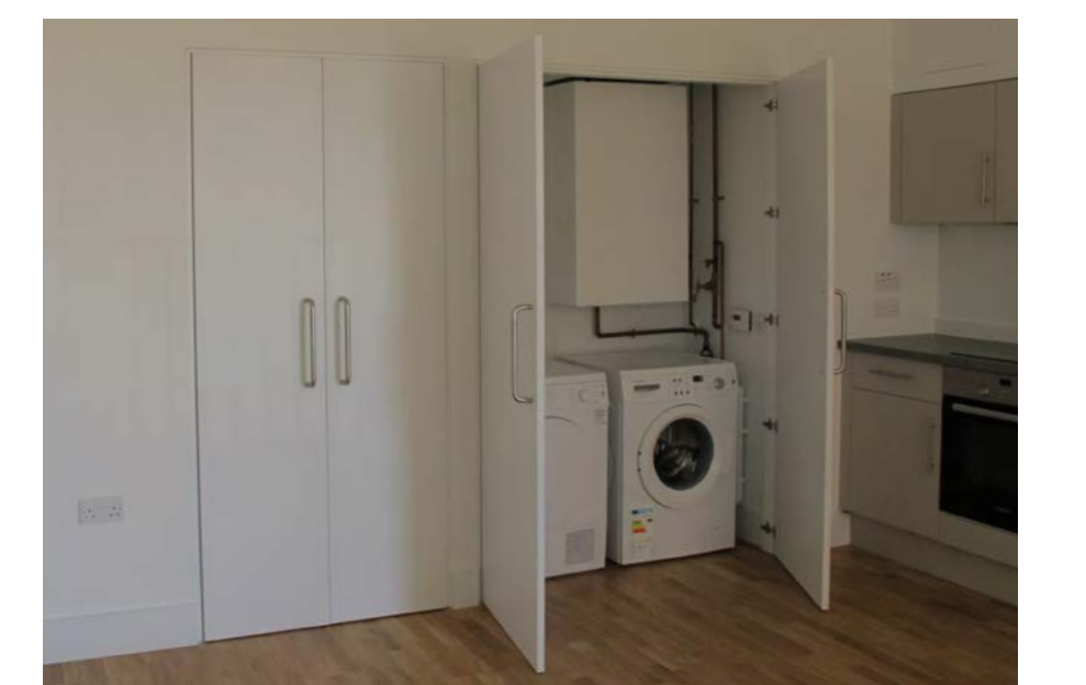
Rationalise storage to work better
