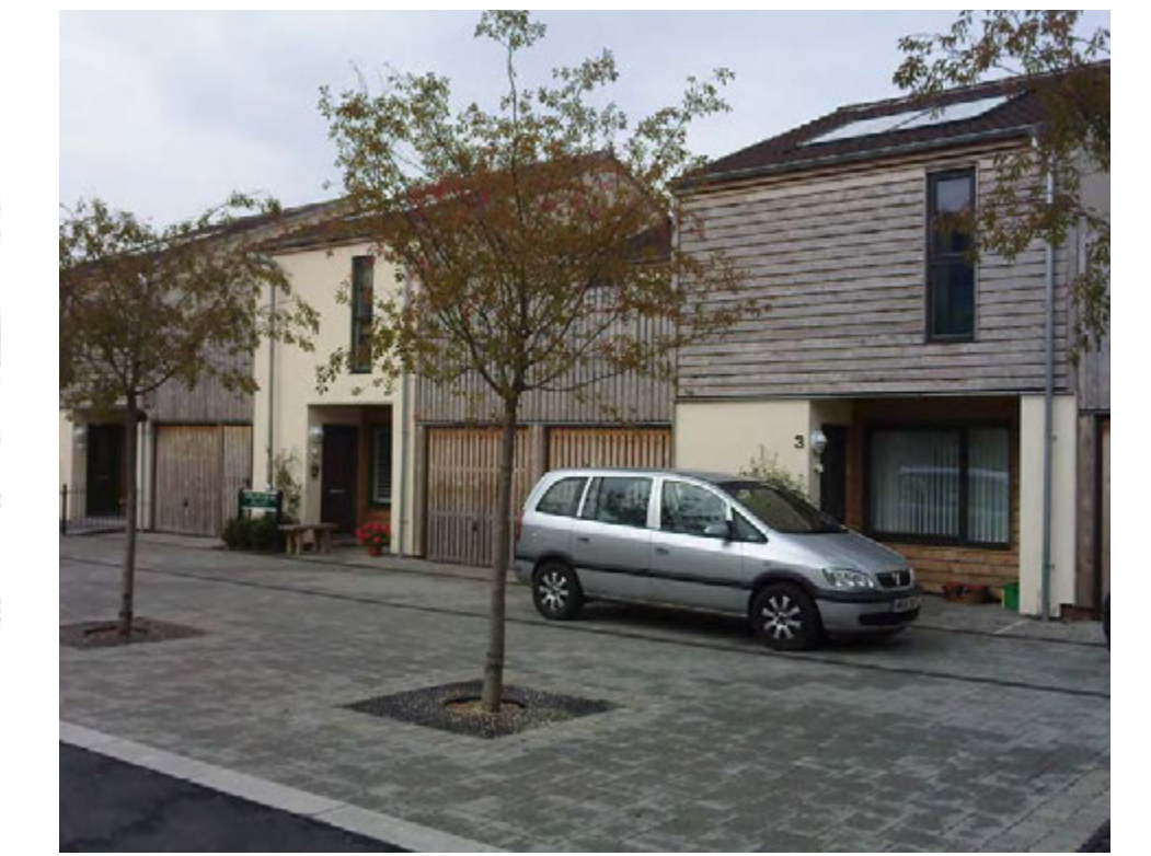
Shared surface with level access to homes
