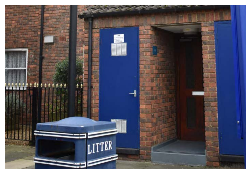
Stepped entrances to flats
