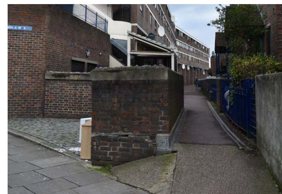
Steep narrow access. Designated area for large rubbish collection.
