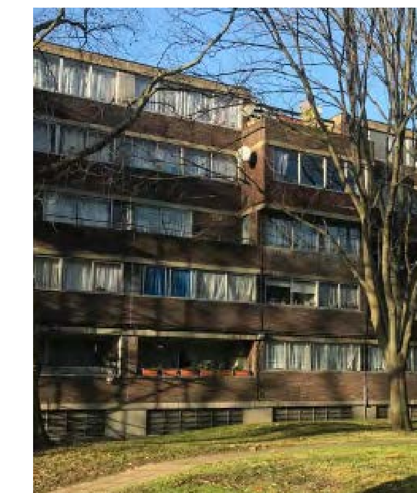
Existing separation of flats from the courtyard
