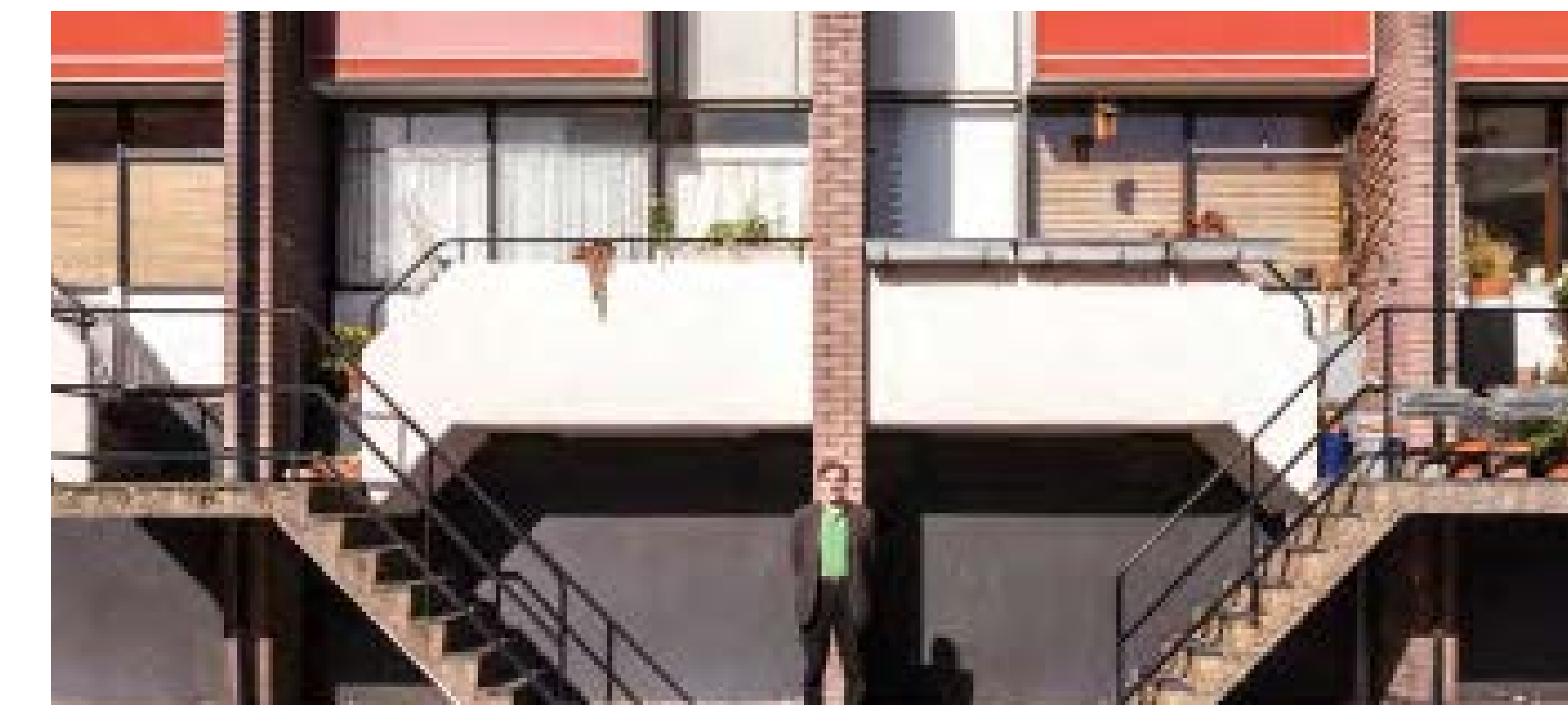
Example of well designed steps to link lower flats to courtyard spaces
