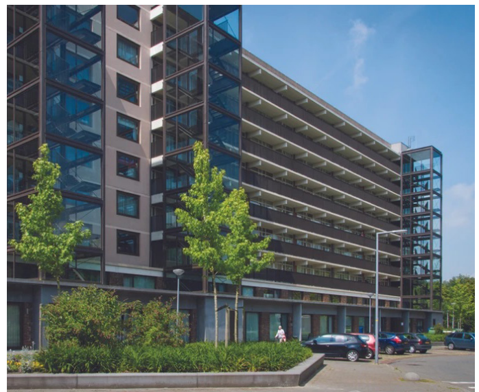
Above and below: HvdHA's Knikflats, Rotterdam. One of the world's leading retrofit projects, the project involved the refurbishment of 1960s-designed homes and communal spaces. The refurbishment included improvements to circulation space, with new cores, lifts and stairs; thermal performance, with new cladding and glazing; and new homes at ground level, creating active, overlooked public realm.
