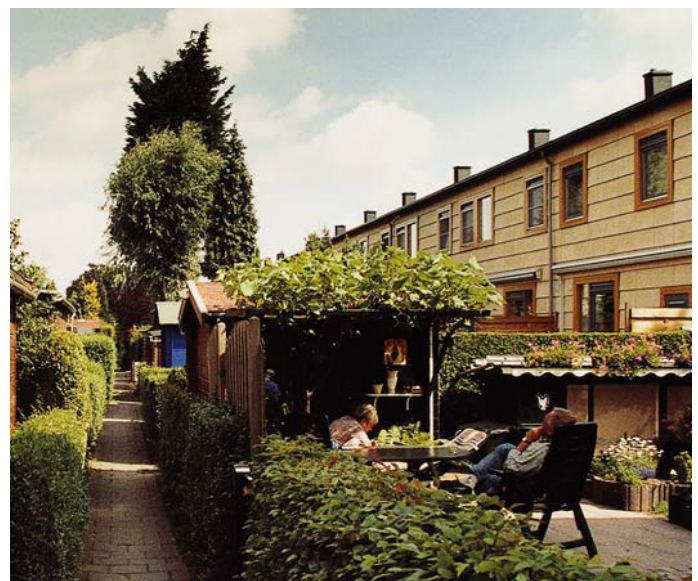
Above: HvdHA's renovation of Tuindorp Kethel, a post-war garden village of 241 low-cost single-family houses built using pre-fabricated construction systems. Rather than demolishing the deteriorated estate, a sensitive refurbishment process was carried out, improving energy efficiency and addressing the needs of individual properties. Residents were involved throughout the renovation process, from the design stage through to the final construction stage.
