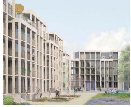
An insulated outer brick skin is being added to the building, with new balconies and stairs down into the communal garden spaces. The skin has completely transformed the appearance of the building, and improved the environmental performance.
