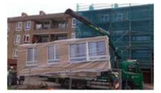
External insulation and prefabricated building elements
