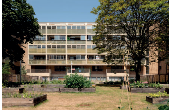
Refurbished buildings with new wintergardens and ground floor apartments which have replaced the old garages
