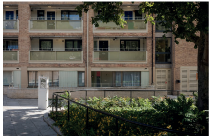
Refurbished buildings with converted garages at ground floor
