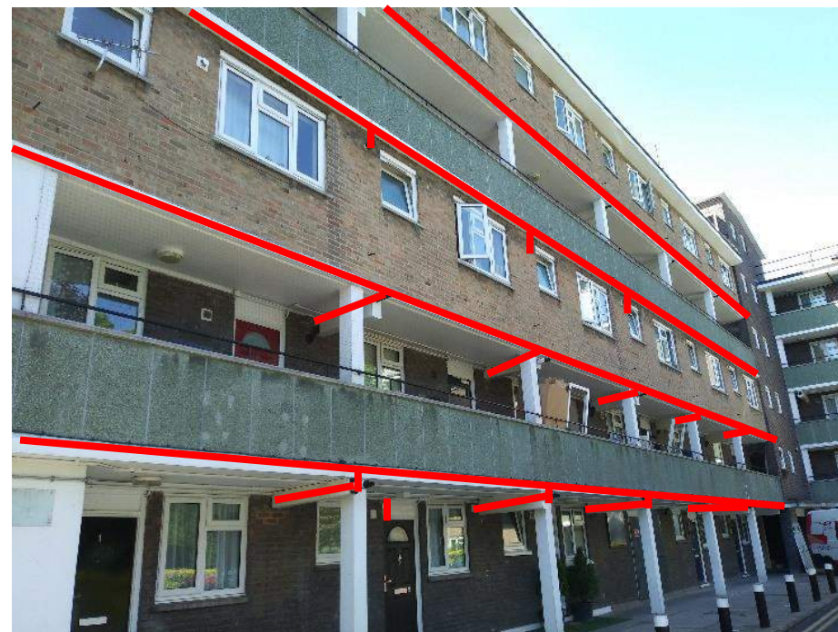
Figure 3.2.14: Pipe connection on the façade – Another view of pipe connection
