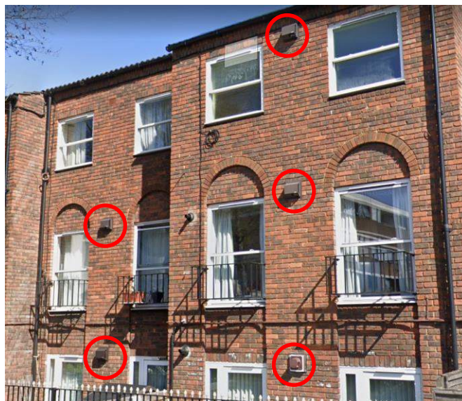
Figure 3.2.9: Top and bottom: Aerial view of the building – Existing boiler flues
