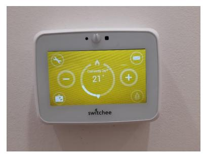
Switchee smart thermostat technology was piloted in this property to test how compatible it is with our existing heating system.
