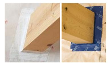
Corners formed around Purlins or Joists are airtightly sealed with Covrum 30/30 or TESCON Profil
