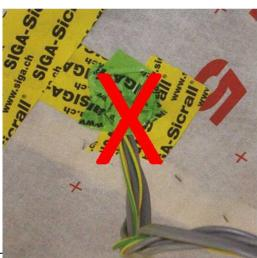
Do not wrap clumps of wires and cables in airtightness tapes as this leaves air gaps between and therfore air leakage.
