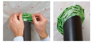
Alternativley, you can use **SIGA RISSAN or pro clima TESCON No. 1** tape to form a cicular airtight seal made up in layers.
