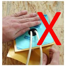
**PRO Clima Kaflex Cable Grommet** enables a better airtight seal for electrical cables that penetrate the airtight seal. Kalflex grommets are manufactured from EPDM which is flexible to form a cicular airtight seal made up in layers. Some **Kalflex** cable grommets feature an integrated adhesive with a release paper for ease of application.
