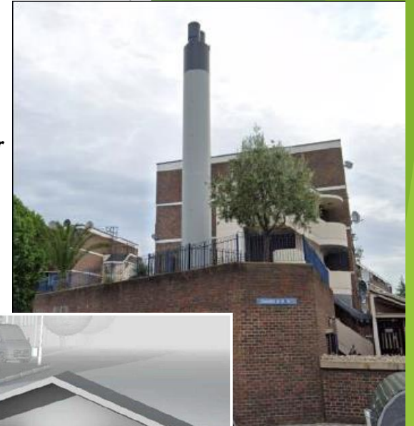
Existing communal boiler
