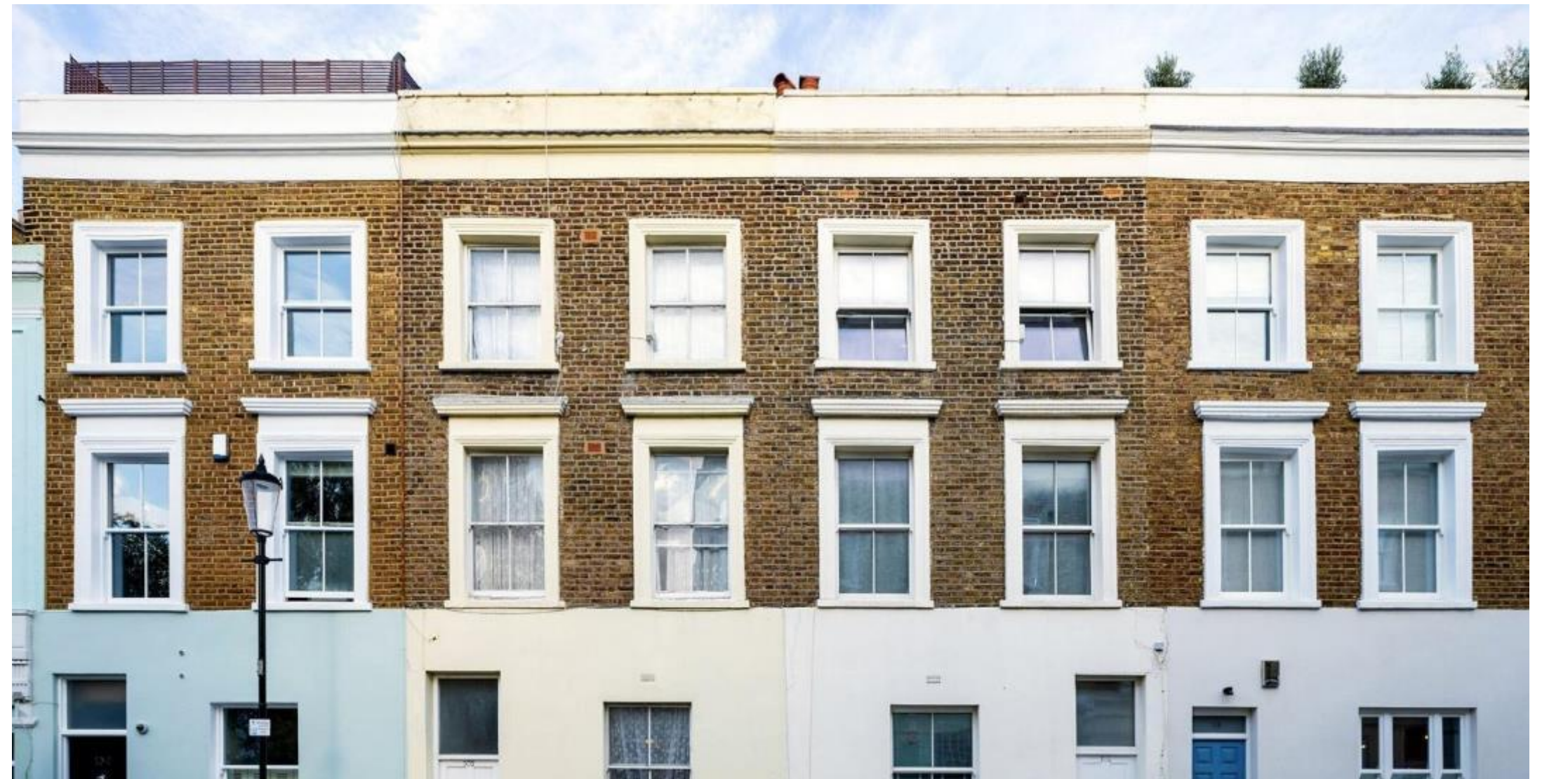
TALBOT GROVE & MORLAND HOUSE
