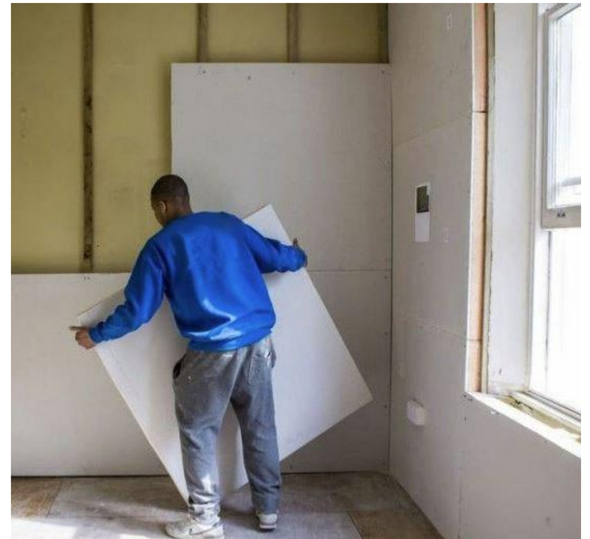
TALBOT GROVE & MORLAND HOUSE
