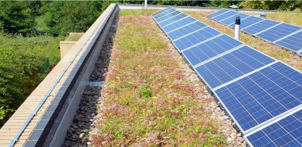
Previous Option 04 - Green Roof + Solar Panels
