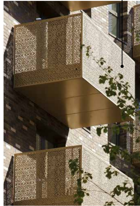
Etched metal to maintain solidity around a balcony without feeling too 'heavy'
