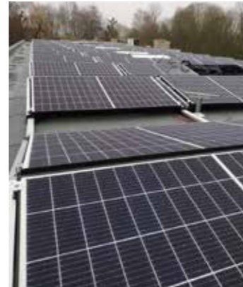
Warm Roof & PVs
