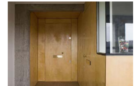
Example of timber front doors
