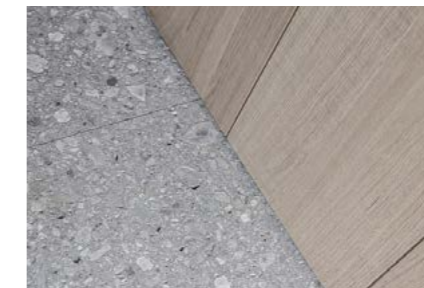
Terrazzo floor & timber doors
