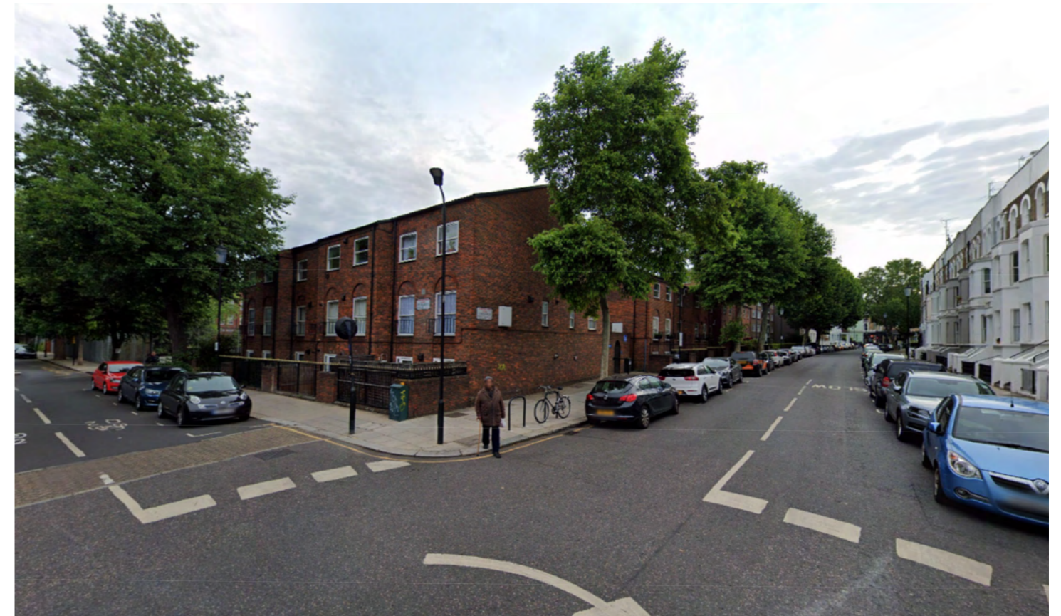
Figure 14 - Camborne Mews view from Cornwall Crescent
