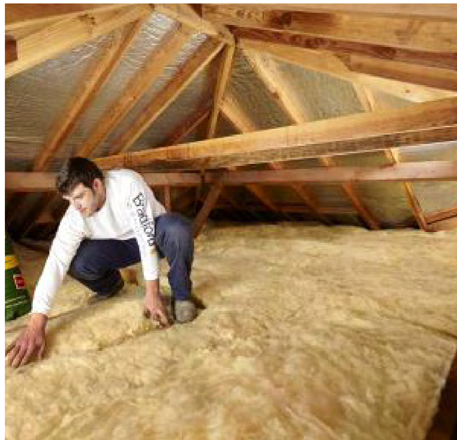
Figure 81 - Mineral Wool Insulation above the existing ceiling joists.
