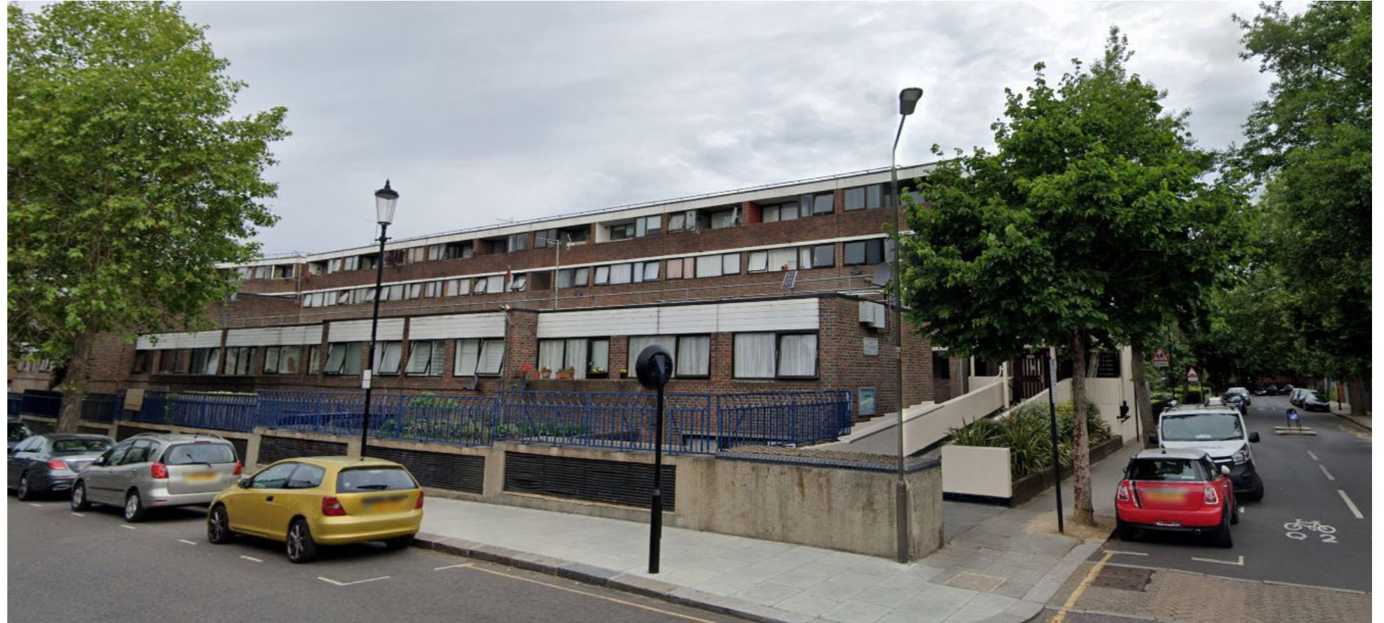
Figure 6 - Camelford Court from Cornwall Crescent
