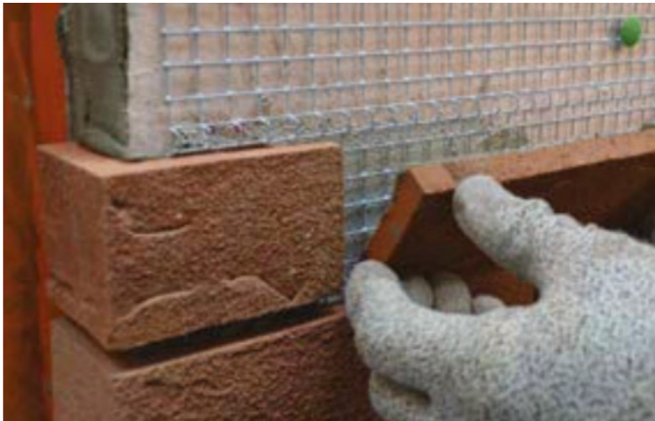
Figure 71 - Brick slips being installed over EWI
