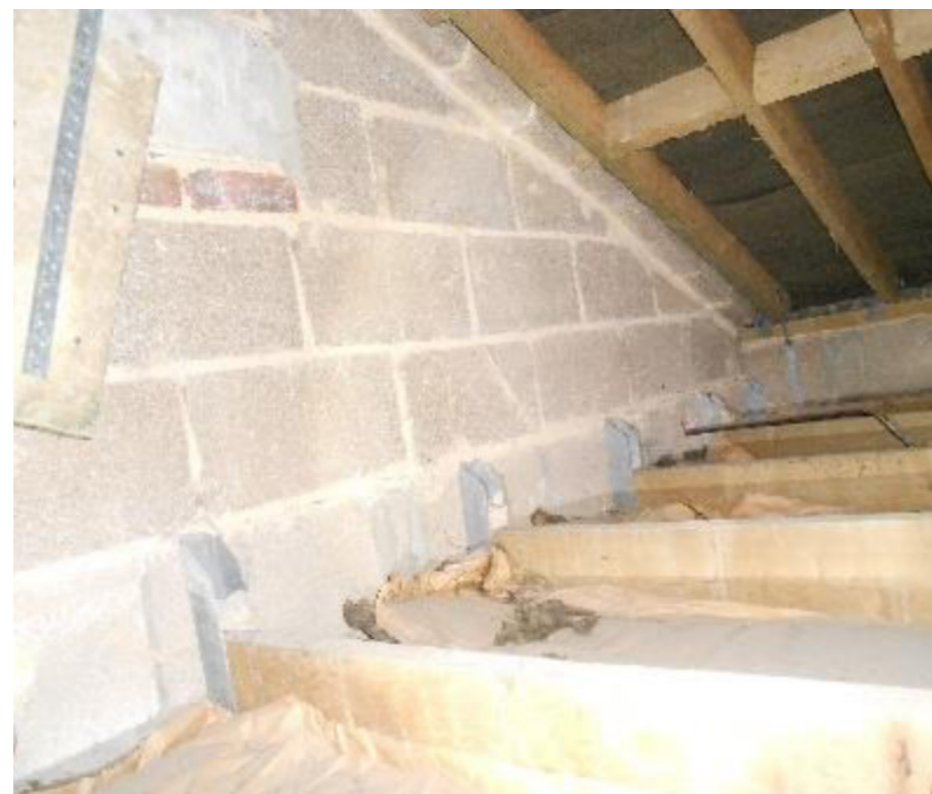
Figure 84 - Existing roof space
