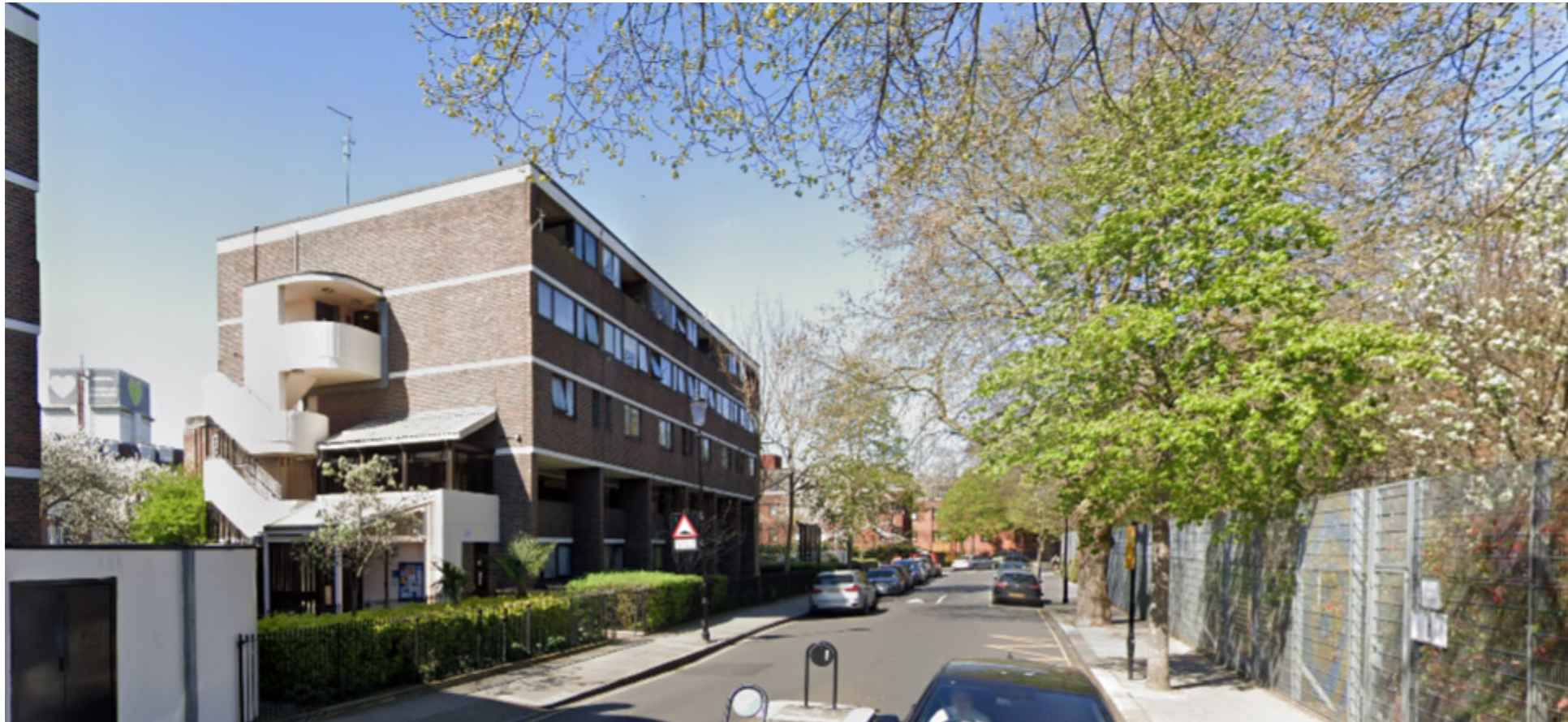
Figure 9 - Talbot Walk from St Marks Road
