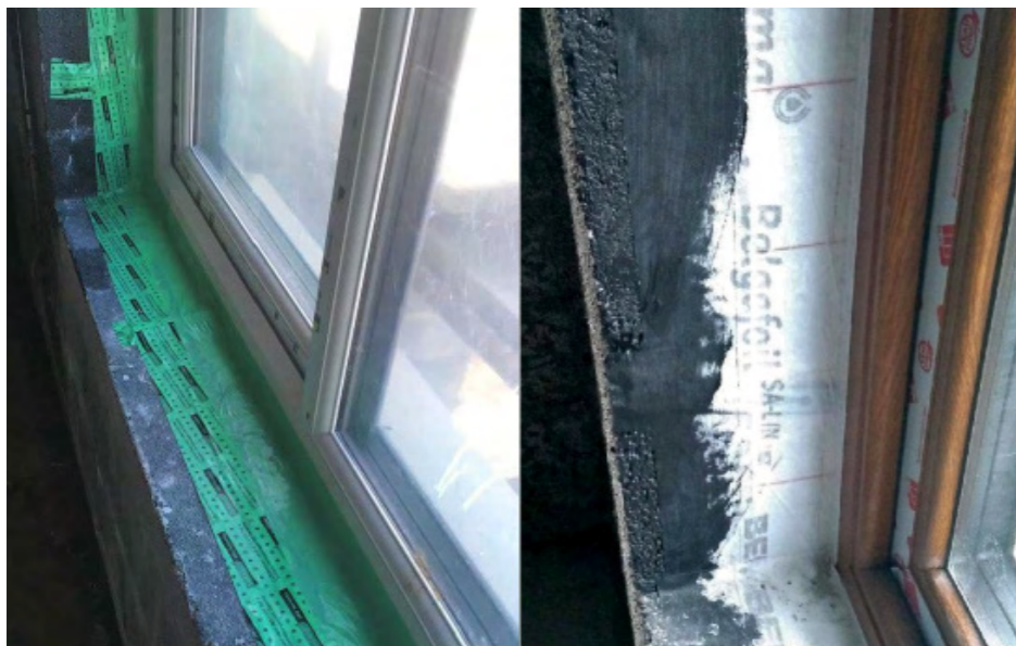
Figure 70 - Airtight window installation
