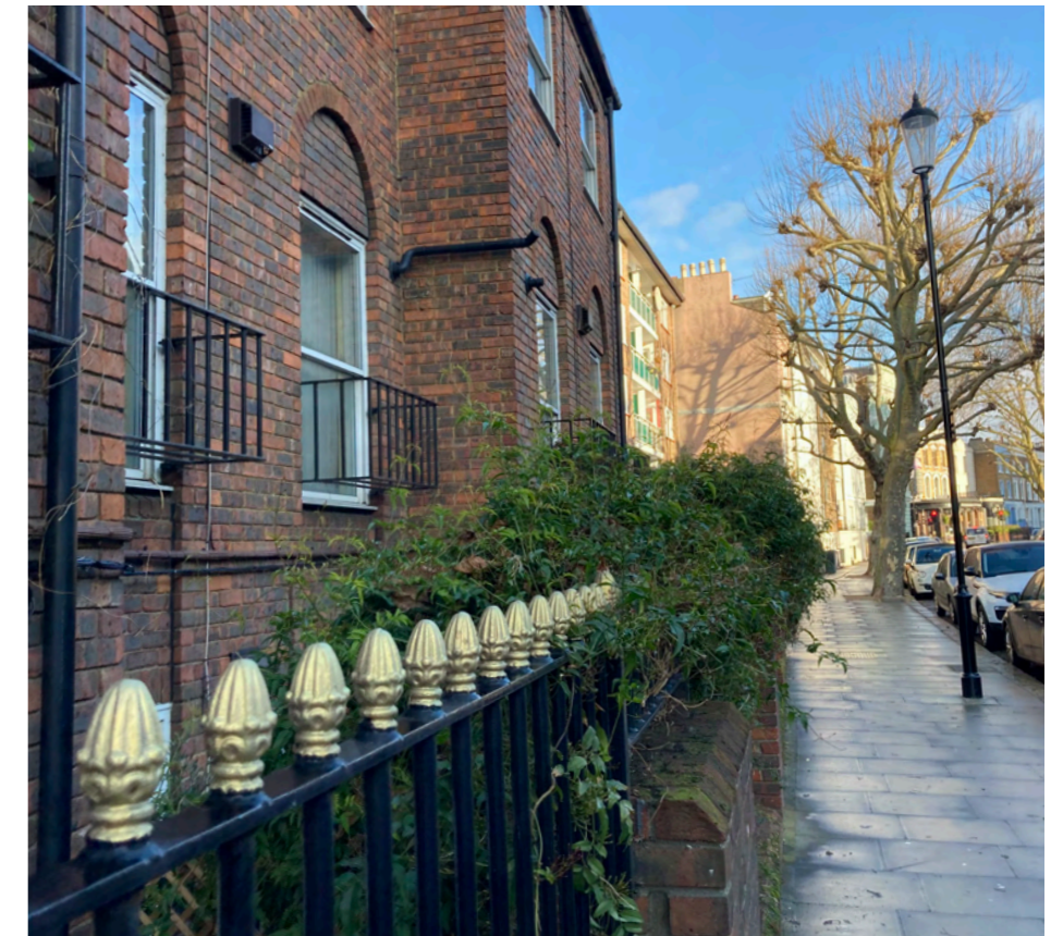
Figure 20 - Rear facade of Cornwall Crescent - balconies and railing detail
