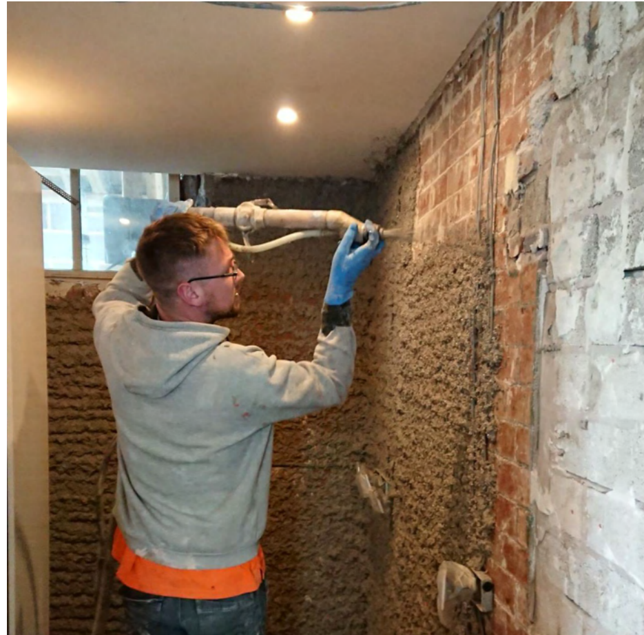
Figure 61 - Woodfibre Insulation added to inside face of external wall.
