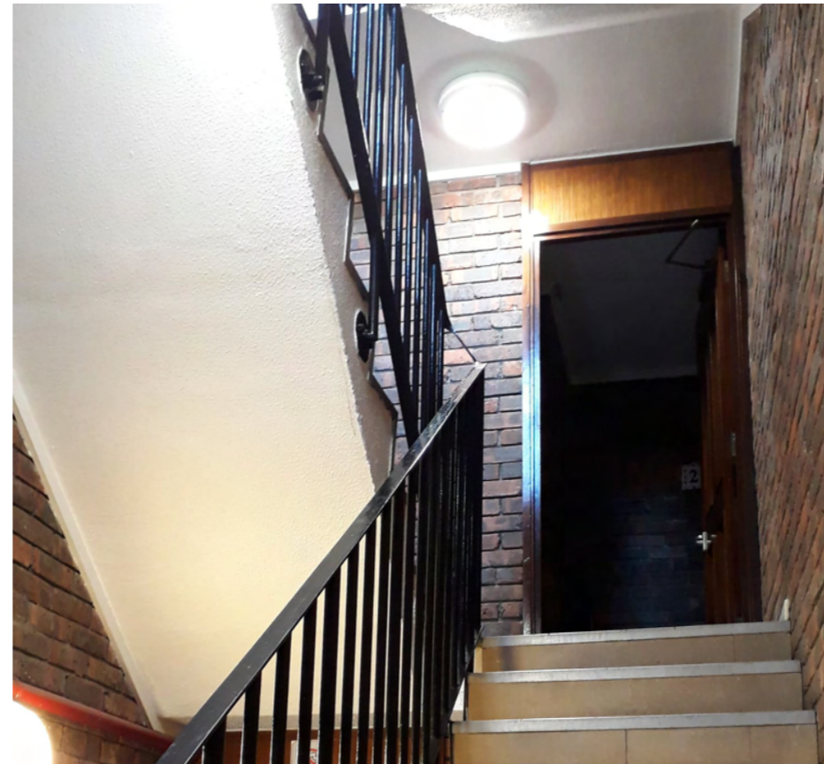
Figure 56 - Reinforced concrete communal stairs
