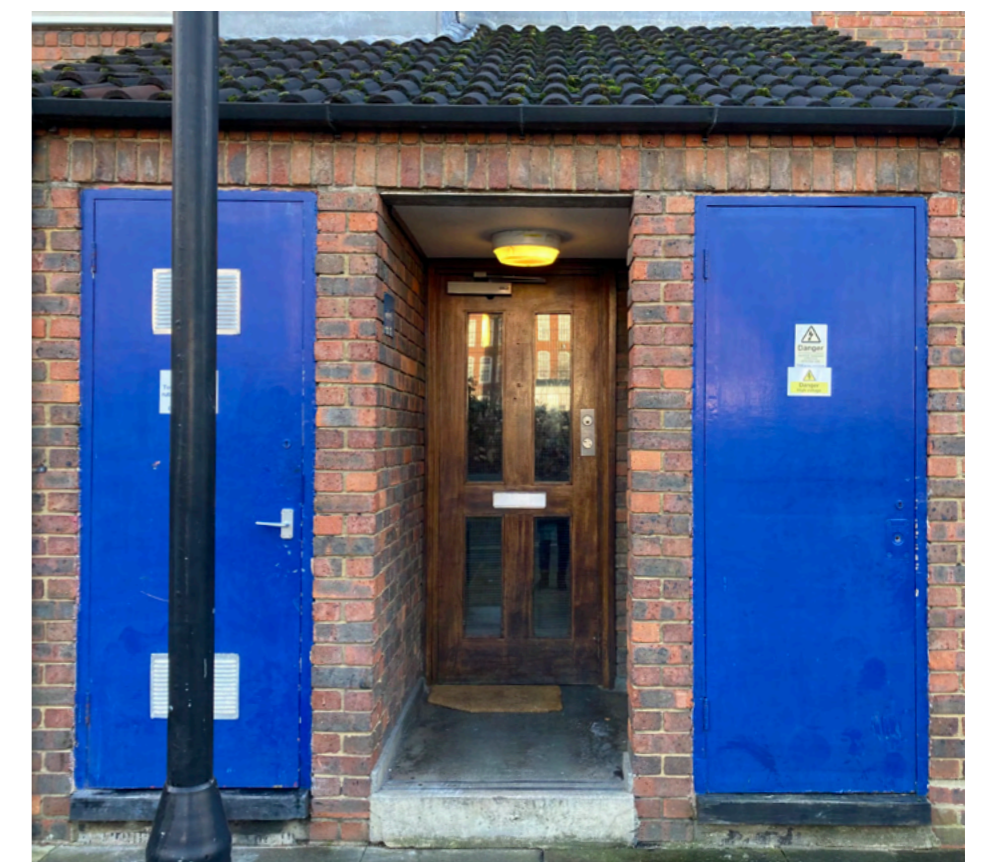
Figure 24 - Existing Control Entry System to access to the Flats
