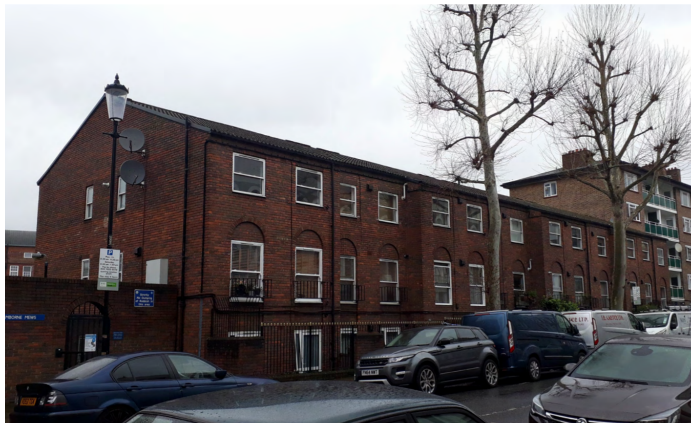
Figure 15 - Camborne Mews view from Cornwall Crescent
