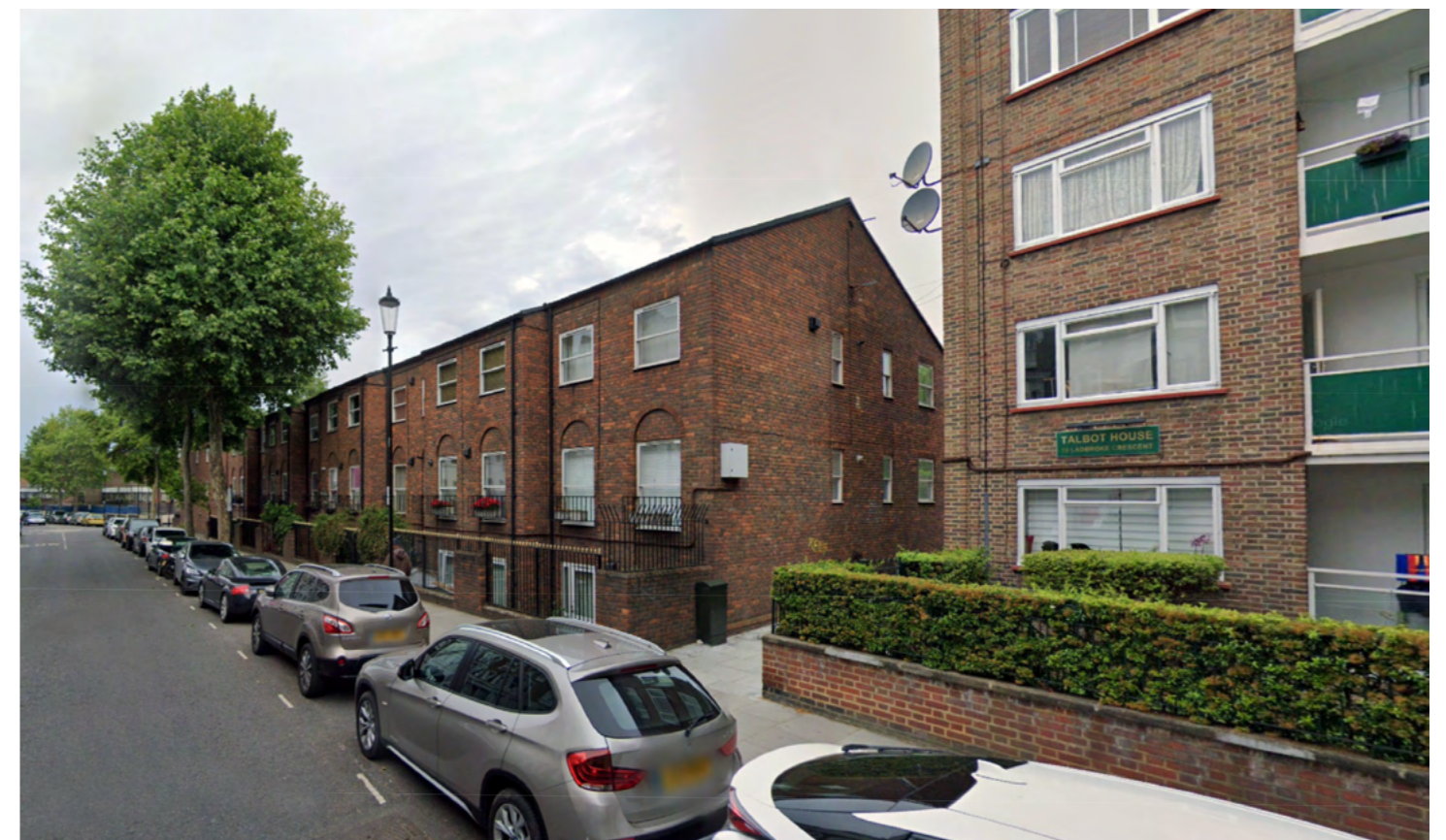
Figure 16 - Camborne Mews view from Cornwall Crescent
