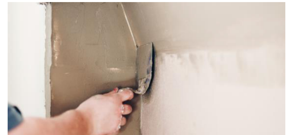
Figure 63 - Aerogel Insulation added to inside face of external wall.
