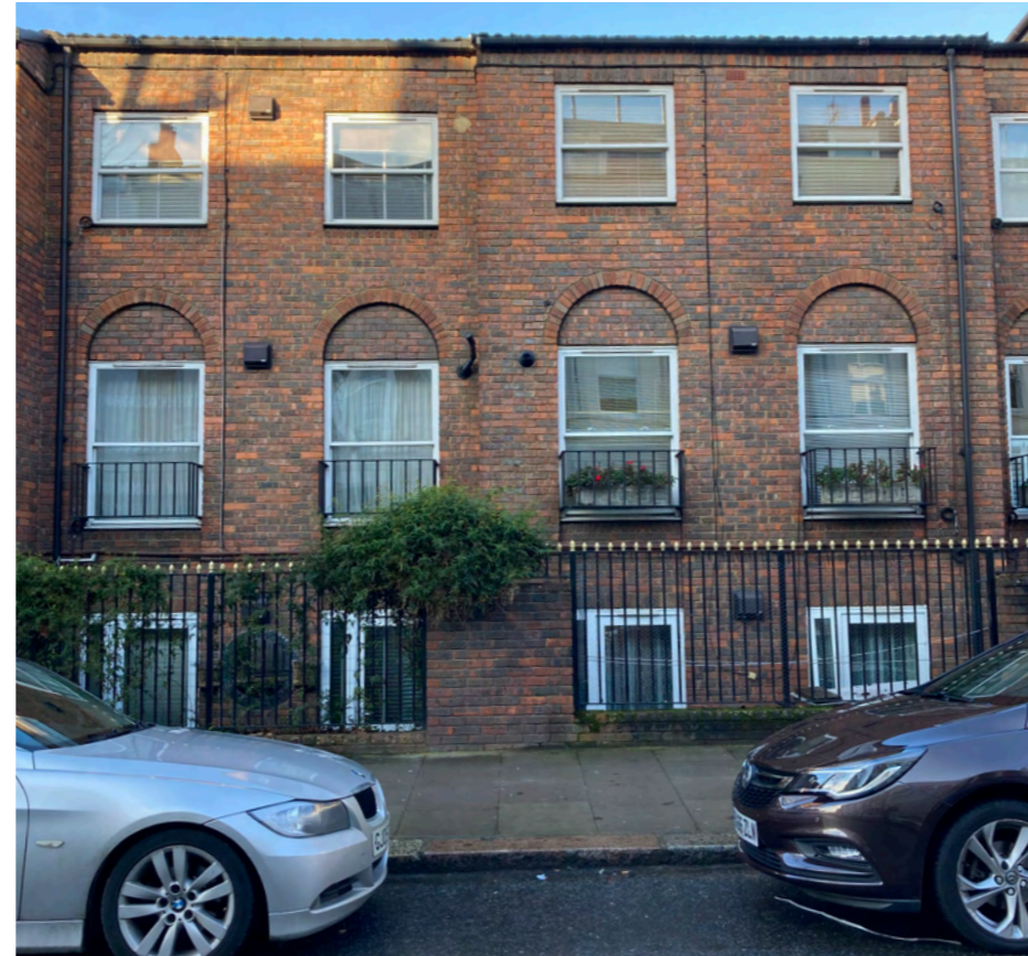
Figure 53 - Ground floor flats below Cornwall Crescent street level
