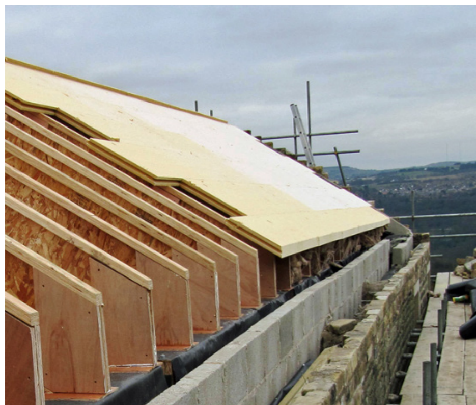
Figure 83 - Insulation added between & over rafters
