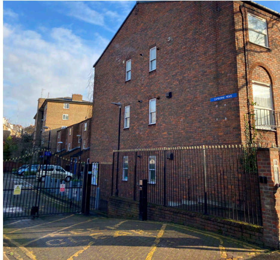
Figure 54 - Sloped ground level from St Marks Road
