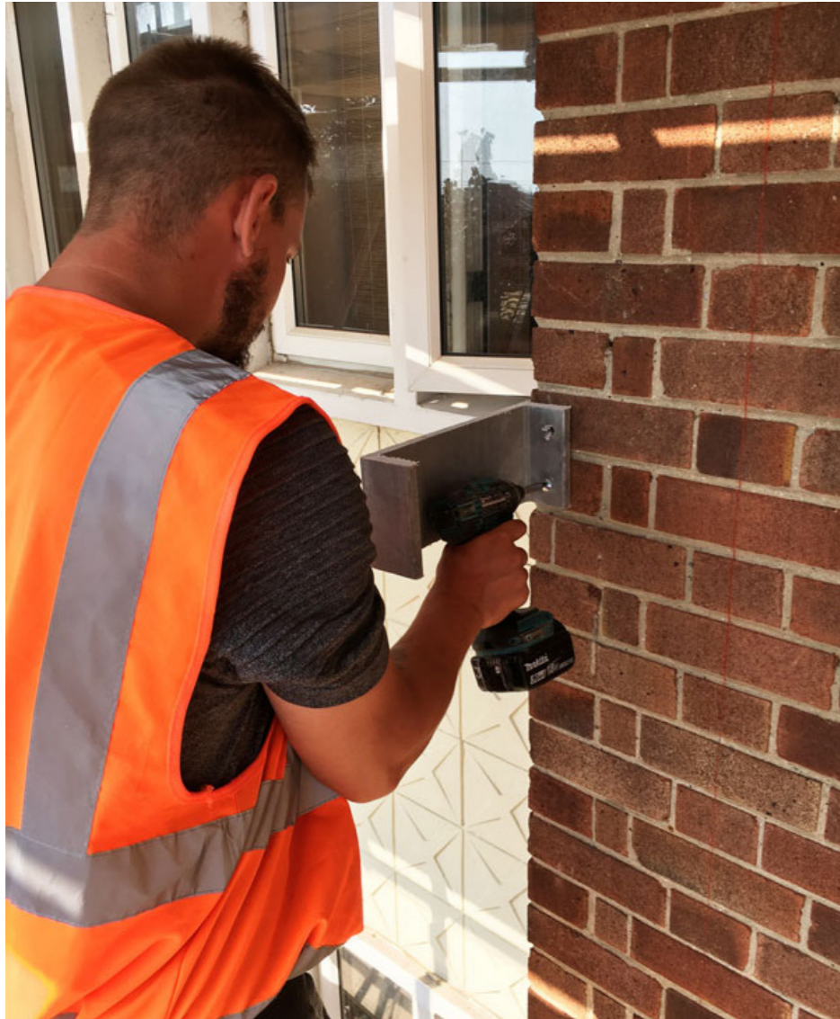
Figure 67 - Beattie Passive system construction process
