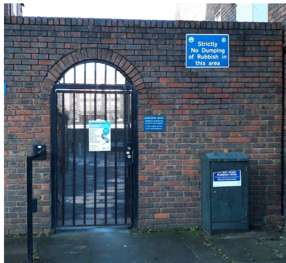
Figure 22 - Existing Pedestrian access from Cornwall Crescent
