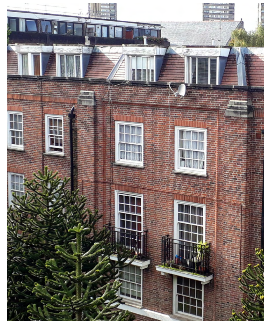
Figure 19 - External facades and fenestration
