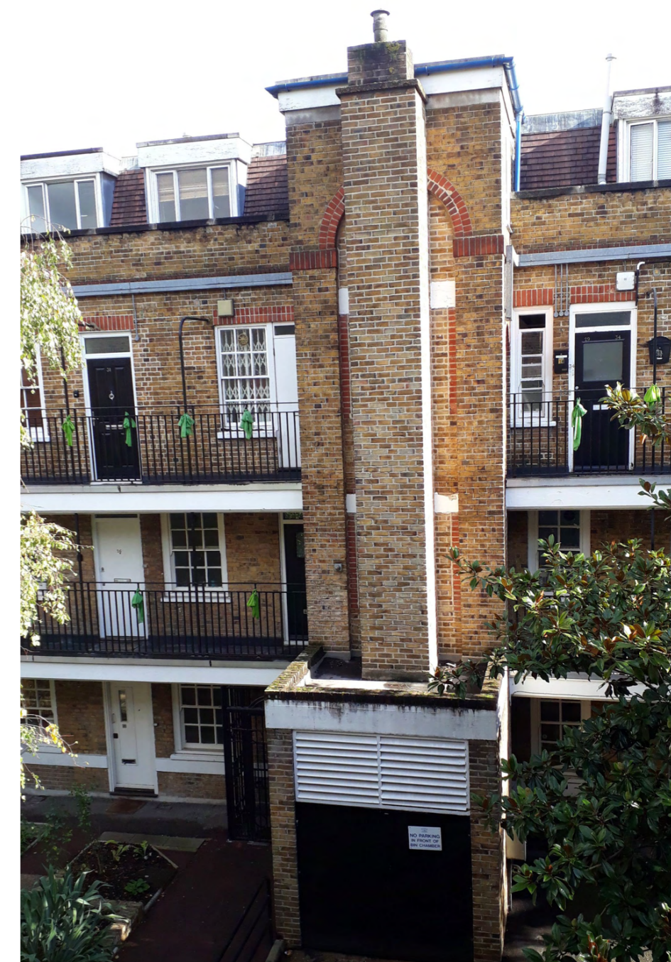
Figure 59 - Morland House. Existing bin chutes, which would need to be altered if lifts are installed in this location
