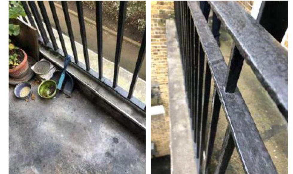
Figure 104 - Condition of existing perimeters
