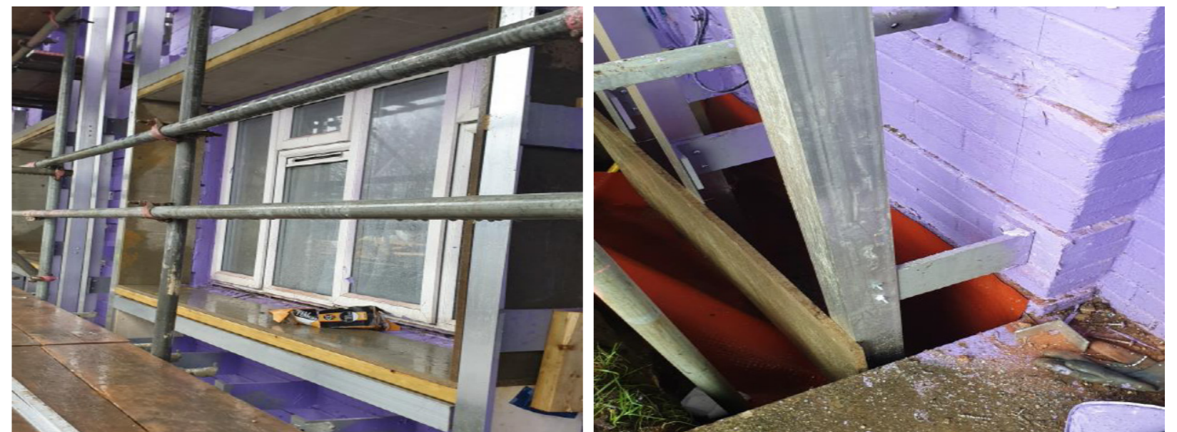
Figure 95 - Beattie Passive system during construction
