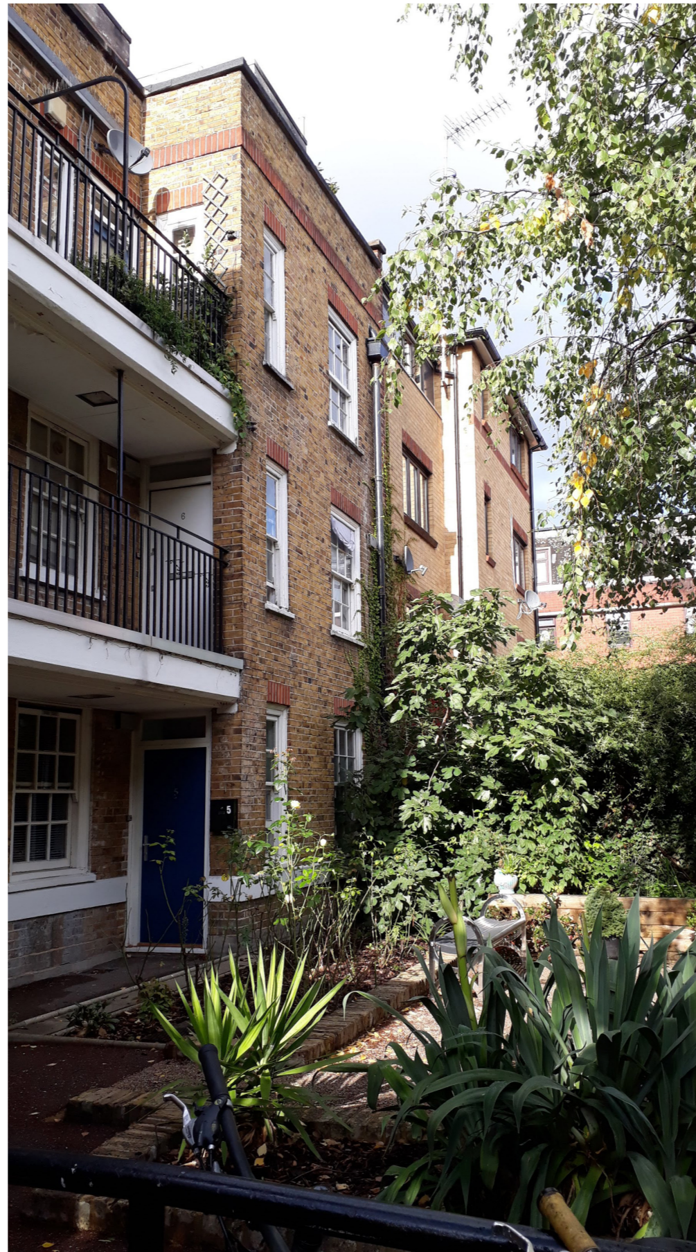
Figure 18 - Internal Courtyard and open walkways
