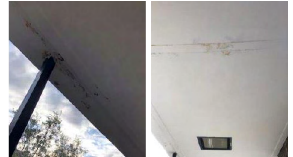
Figure 106 - Condition of existing roof areas
