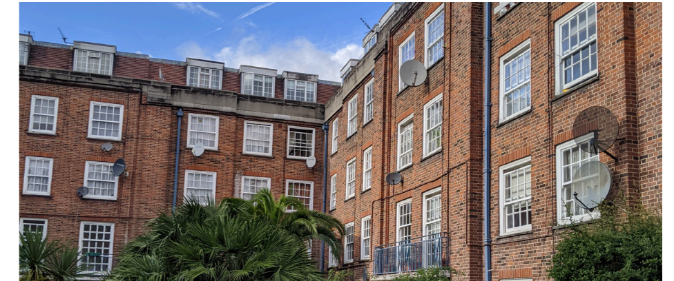
Figure 14 - Talbot Grove House
