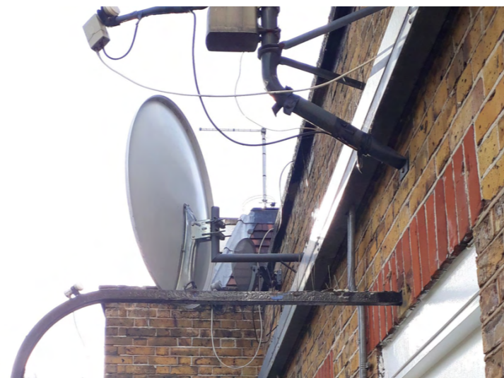
Figure 58 - Morland House. Existing aerials on walkways
