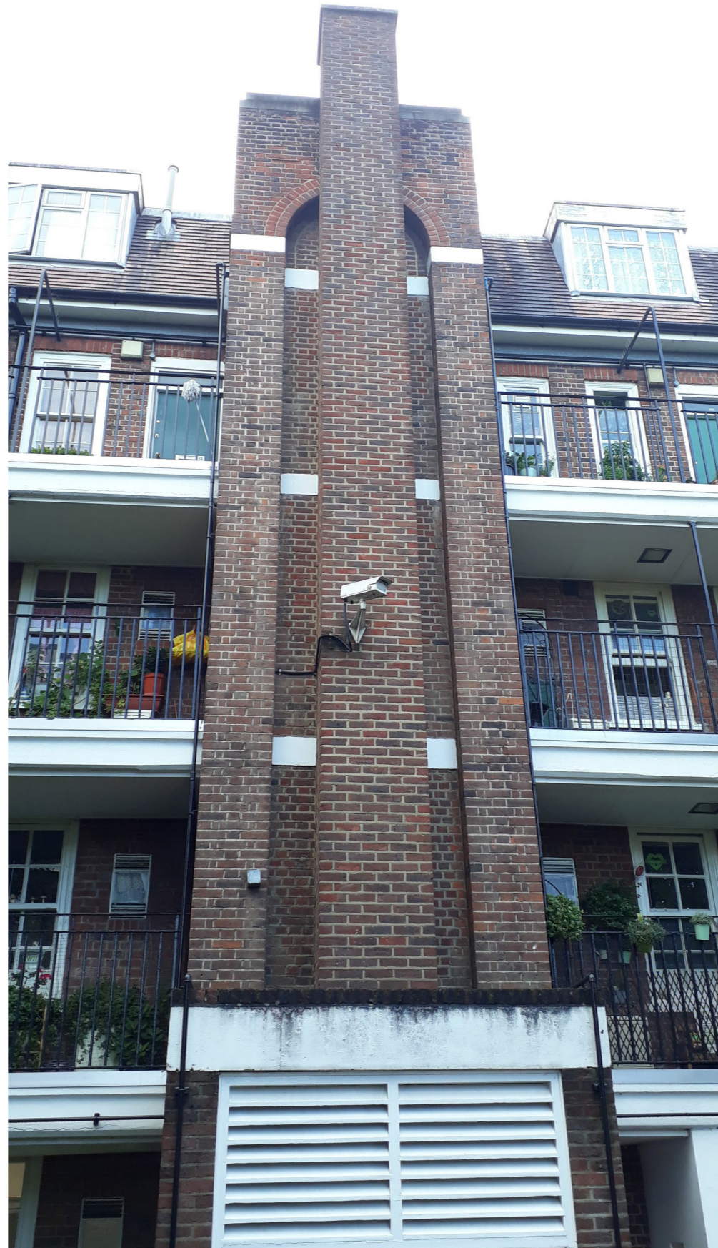
Figure 29 - Existing Bin Chute
