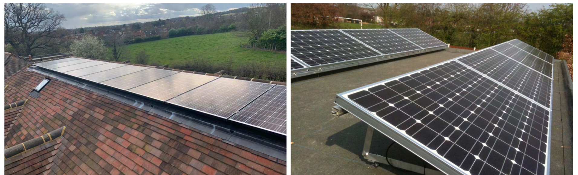
Figure 101 - Types of PVs mounted on flat roofs
