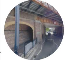
Narrow pedestrian passage under the railway bridge
