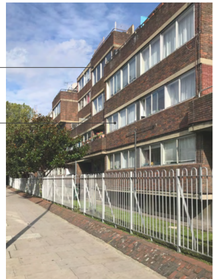
Possible areas of focus for external envelope works
