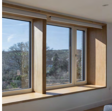
Composite windows provide an opportunity for a timber internal finish for warm softer appearance
