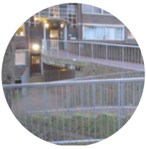
Elevated access is secured by railings
