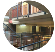
Access to the flats from the upper walkway
