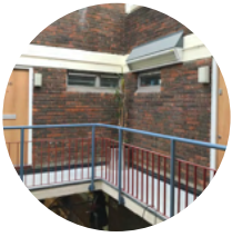
Upper level bridge access to homes
