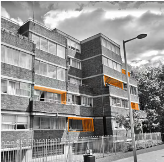
Sketch studies considering the thermal improvement and lining of entrances and individual balconies to provide entrance legibility (Gbolade Design Studio)
