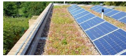
Option 4: Green Roof + Solar Panels
