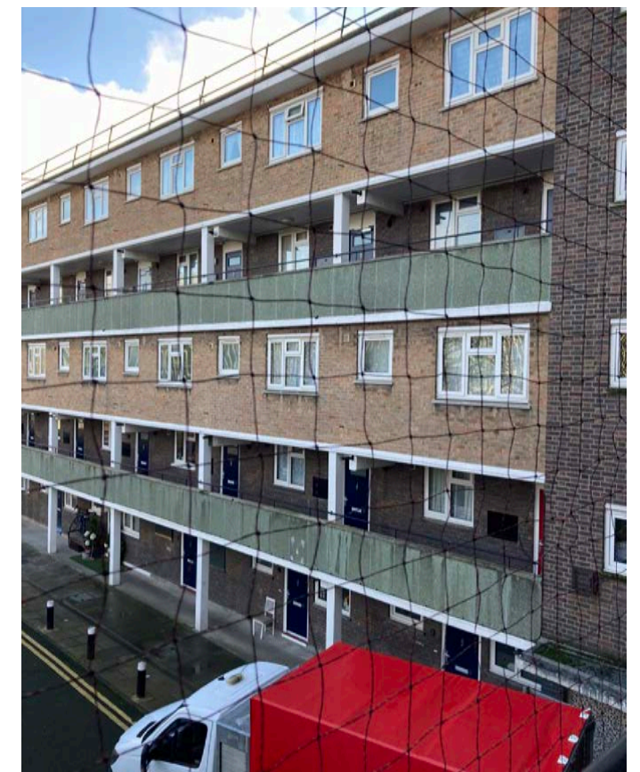
6 Treadgold House north facade
