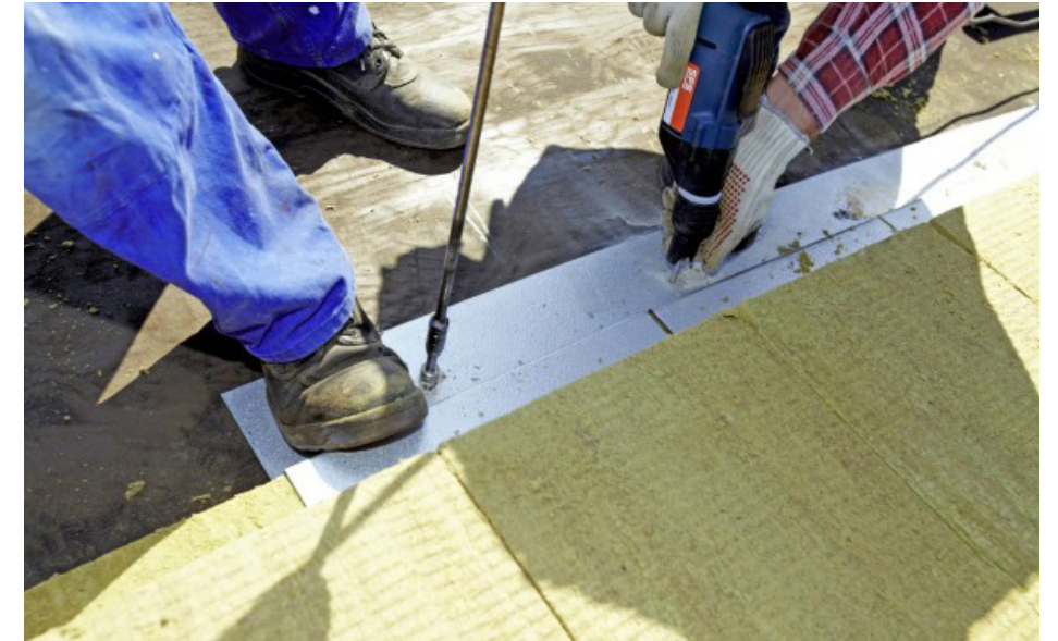
Figure 48 - Mineral wool insulation being installed on a roof
