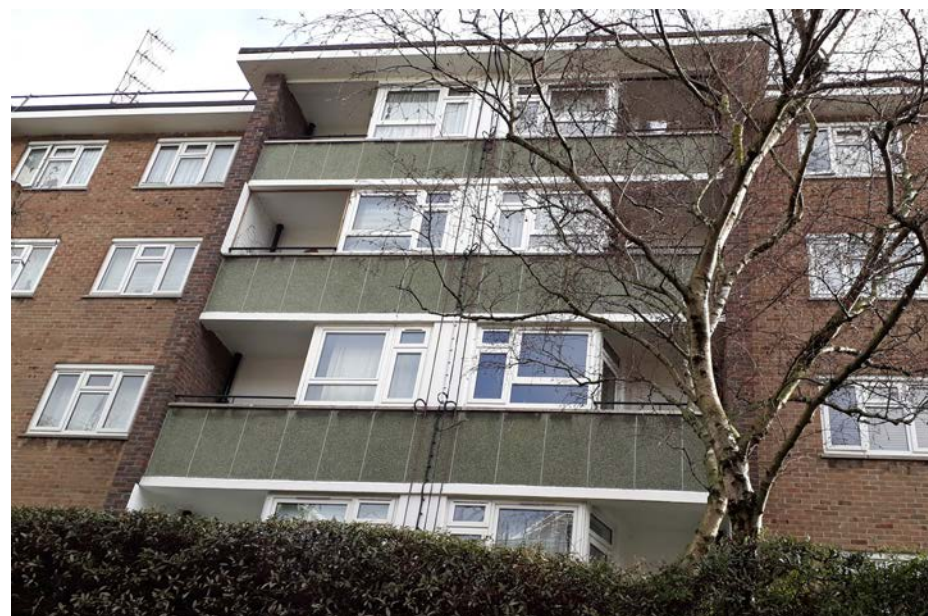
Figure 25 - Rainwater pipes run down rear corner of inset balconies
