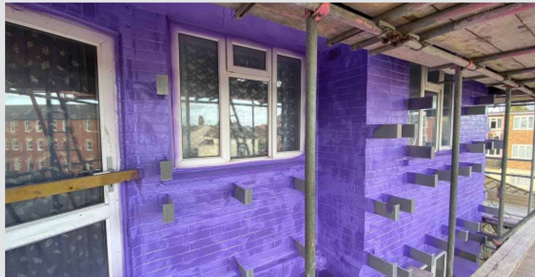
Figure 40 - Beattie Passive system construction process
