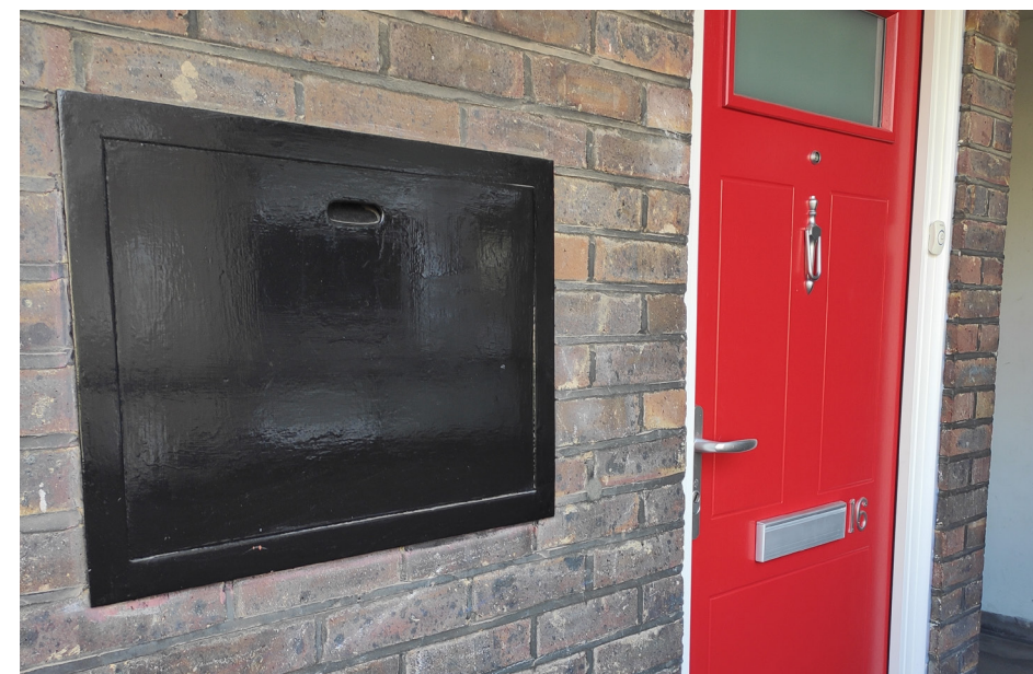
Figure 28 - Coal chute door
