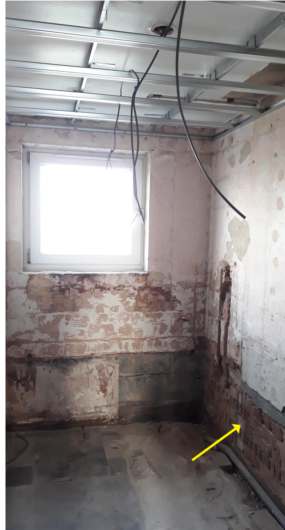
Figure 13 - Brick separating walls
