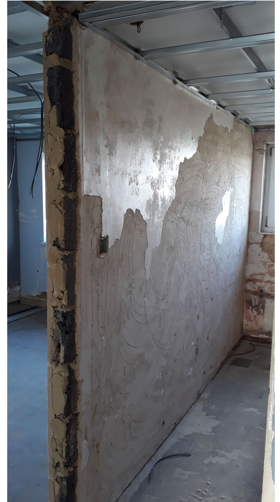
Figure 14 - Block work internal partitions
