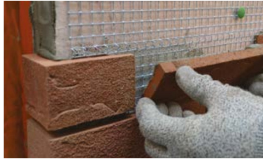
Figure 35 - Brick slips being installed over EWI
