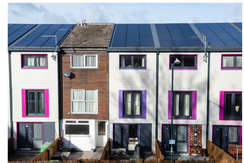
Figure 41 - Melius Homes Modular completed retrofit schemes
