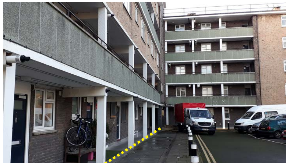
Figure 11 - Assumed Concrete foundation edge line (view from the car park)
