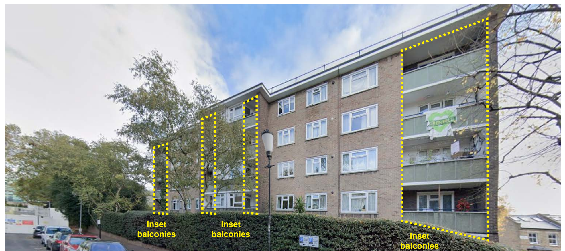
Figure 8 - West wing - West facade
