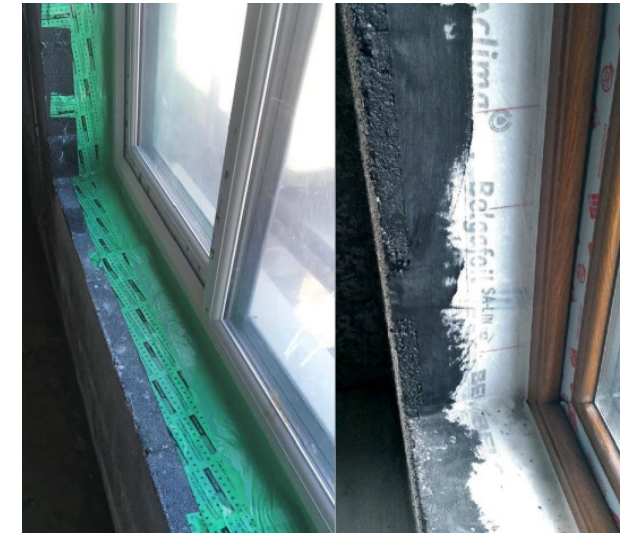
Figure 37 - Airtight window installation
