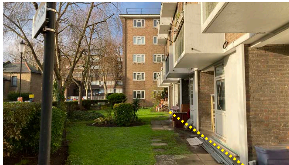
Figure 12 - Assumed Concrete foundation edge line (view from the main gate)
