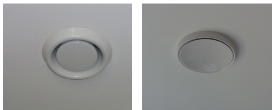
Figure 58 - Ceiling mounted air supply and extract valves
