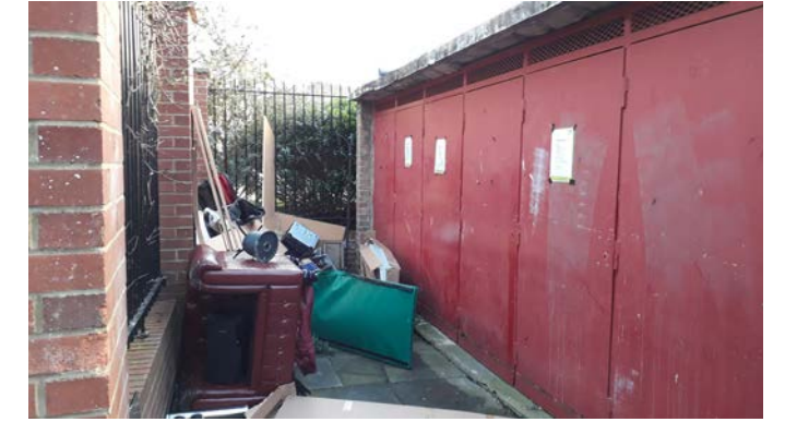
4 Storage spaces adjacent to the main gate
