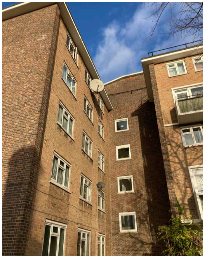
2 Treadgold House staircore from Bomore Road
