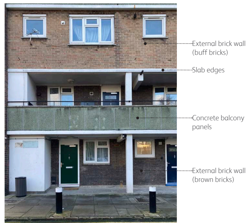
Figure 9 - East wing - North facade
