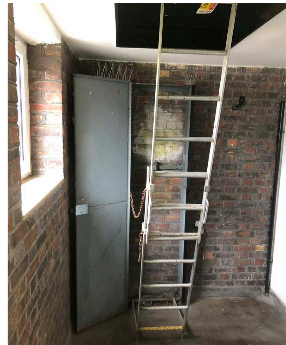
Figure 15 - Access to the roof from the third floor
