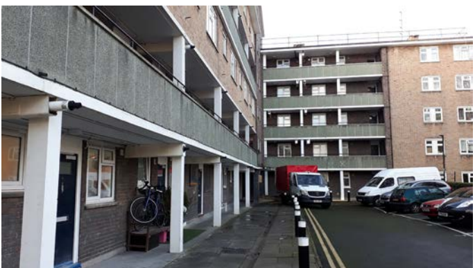
3 Treadgold House car parking
