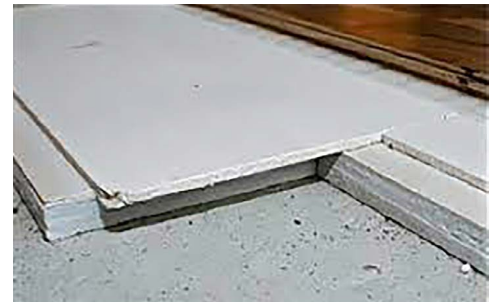
Figure 47 - Aerogel insulation with Magnesium Oxide Board
