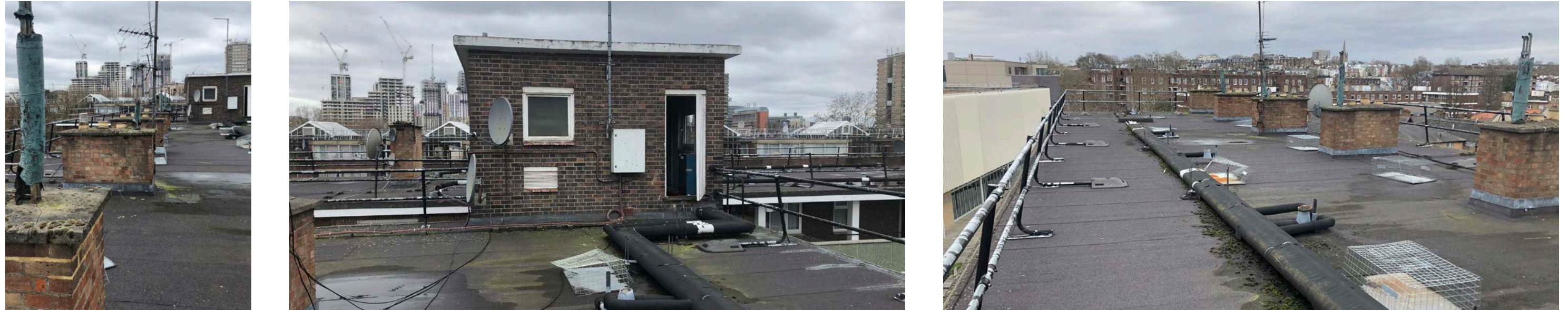
Figure 18 - East wing roof conditions
