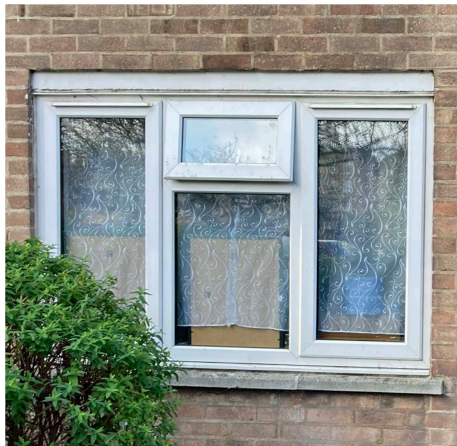
Figure 42 - Existing typical window divided in 4 parts
