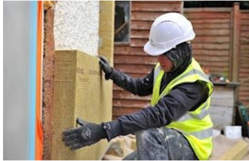
Figure 36 - EWI construction process
