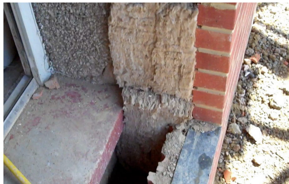
Figure 46 - Insulation 'skirt' being installed below ground
