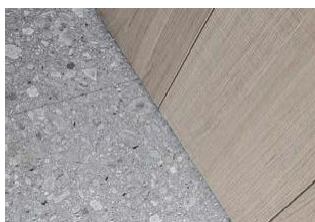
Terrazzo floor & timber doors
