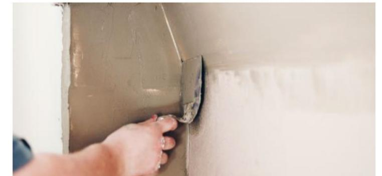
Aerogel Insulation added to inside face of external wall
