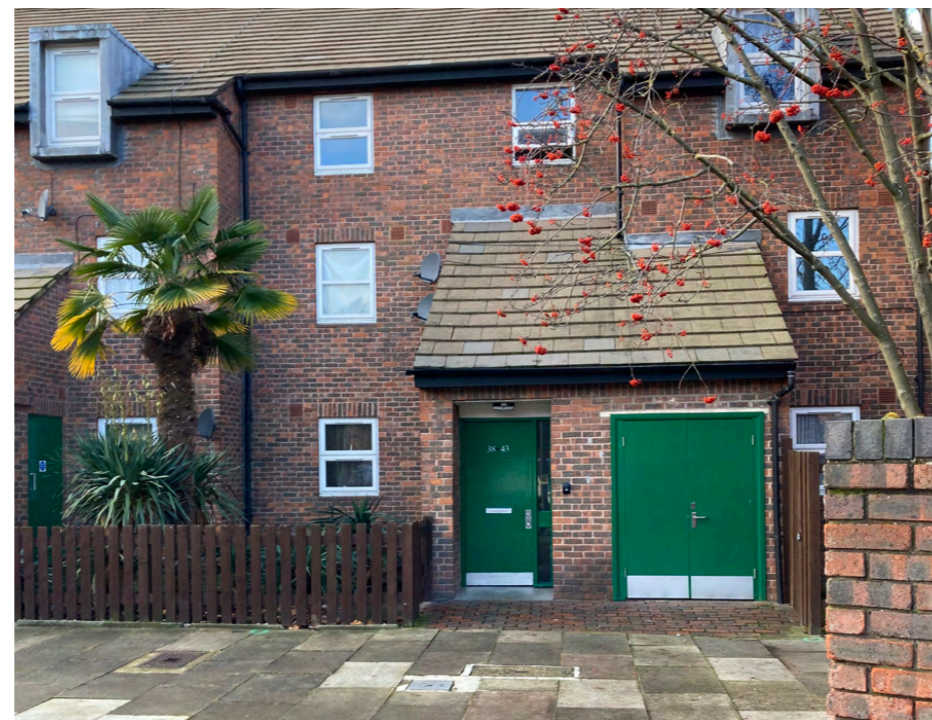
Figure 95 - Existing entrance area to one stairwell of the flats
