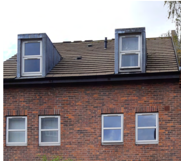
Figure 21 - Dormers to second floor of houses
