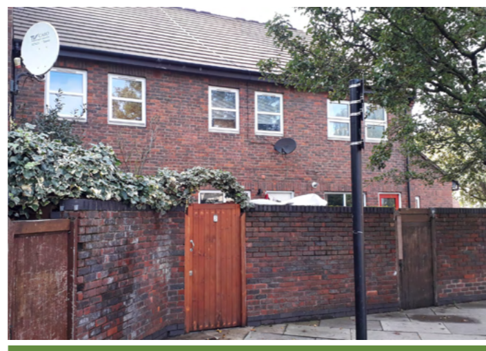
2 storeys to 'front' 1.7m high brick wall
