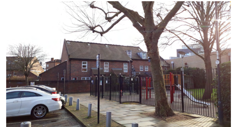
Figure 89 - View of playground fencing where some refuse stores are suggested
