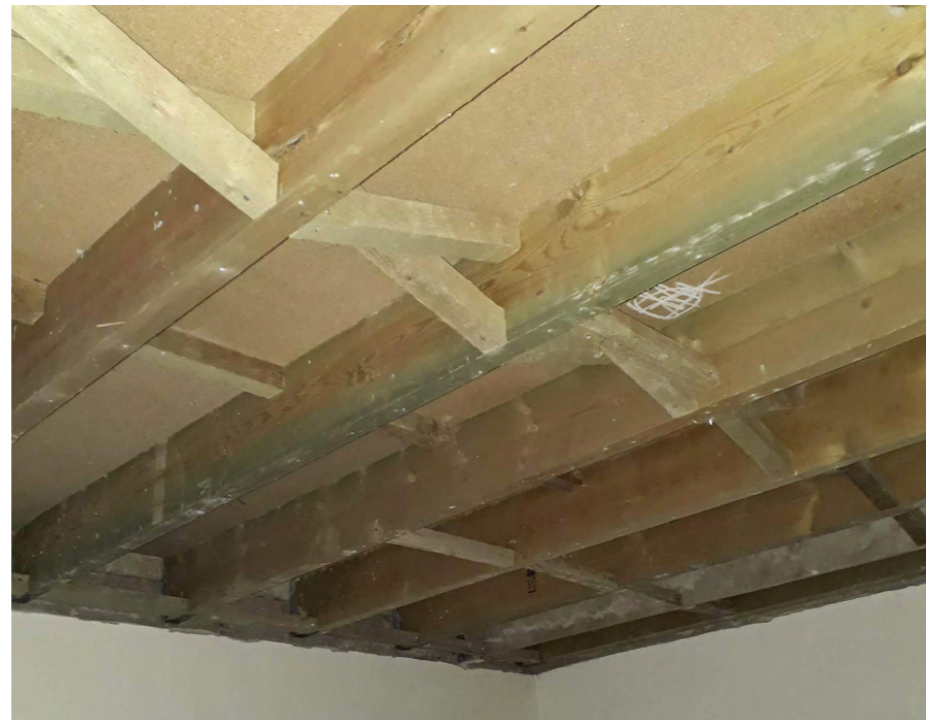
Figure 77 - Existing first floor joists and strutting at 50 Verity Close
