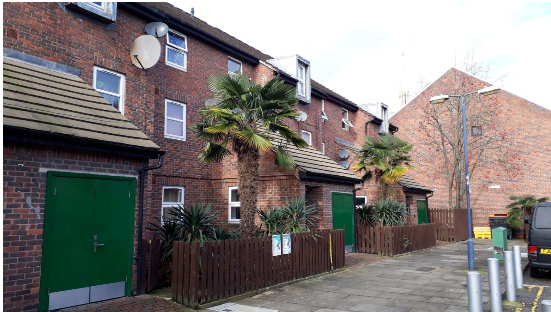
Figure 83 - Currently bin stores (green double doors) dominate front of flats. Loose recycling bin sitting by gable end of house
