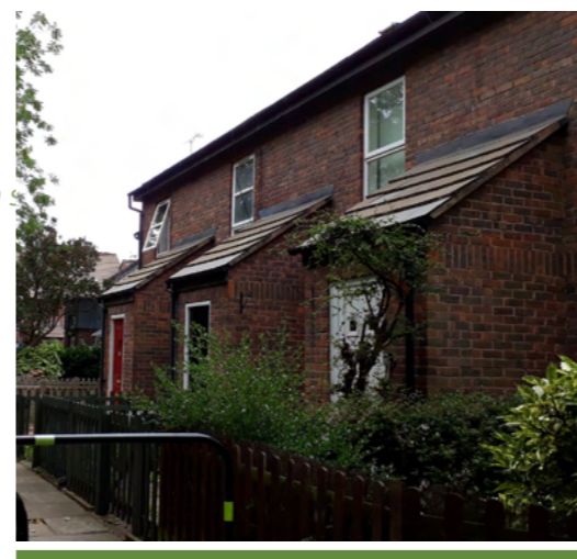
2 storeys to 'rear' Lean-to rear entrances Lower fence to rear
