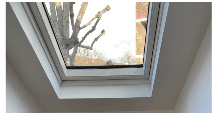
Figure 66 - New triple glazed rooflights at 50 Verity Close. These examples are made by Velux, and can function like other Velux rooflights
