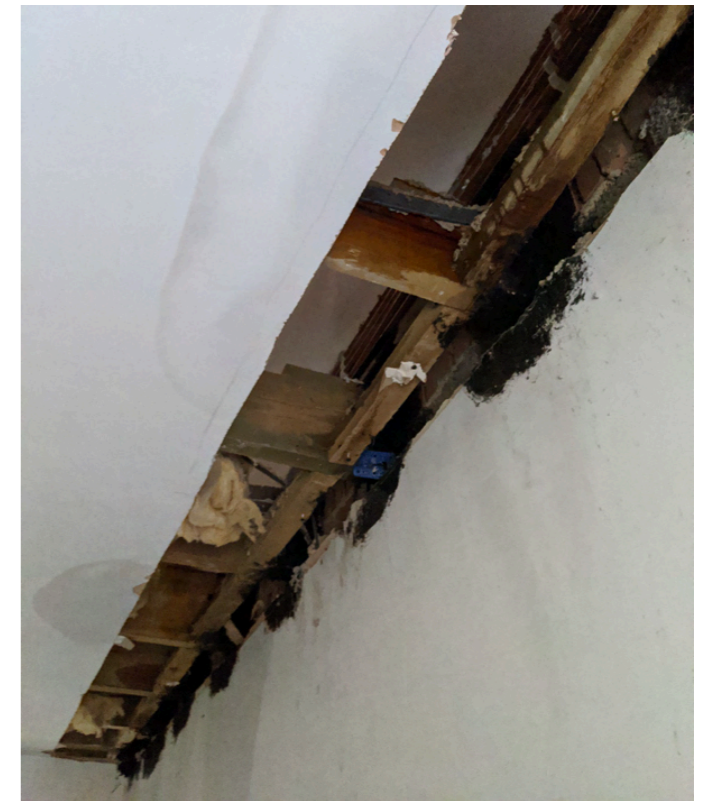
Figure 31 - 50 Verity Close - joist ends exposed & made airtight
