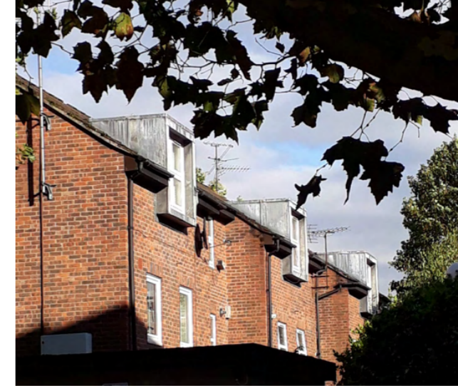
Figure 23 - Larger rear dormers to flats, breaking the eaves line
