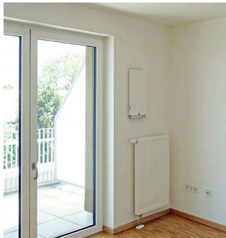
Figure 57 - Through-wall unit installed (the box above the radiator)
