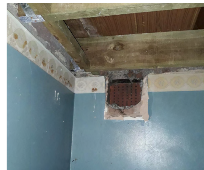
Figure 16 - Vents through walls
