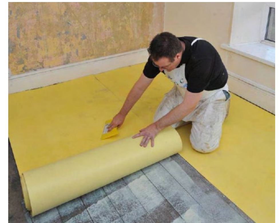
Figure 81 - New resilient mat being fitted over floorboards
