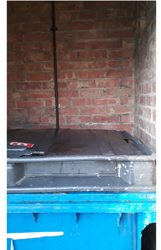
Figure 84 - Inside existing bin store
