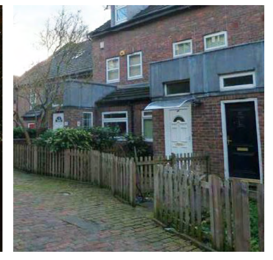
2.5 storeys to 'rear' Dormer to rear Extended rear lobby & lean-to Lower fence to rear
