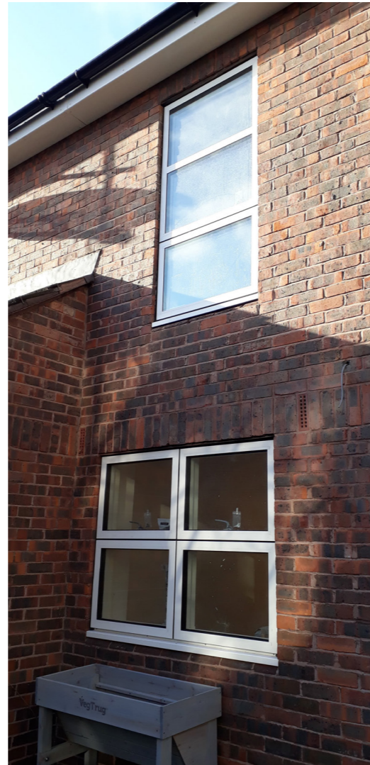
Figure 64 - New triple glazed windows at 50 Verity Close
