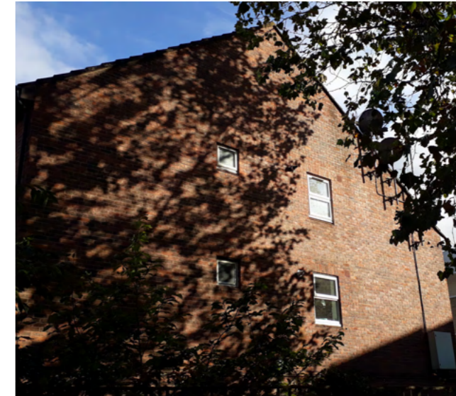
Figure 24 - Windows to gable ends of flats
