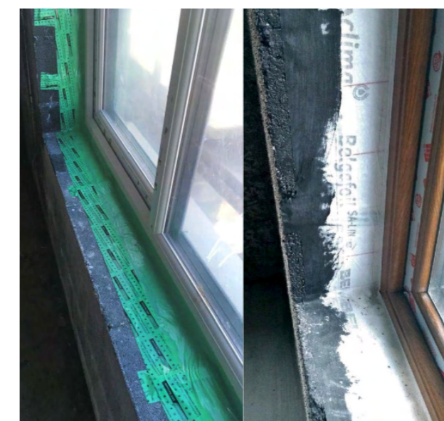
Figure 47 - Airtight window installation
