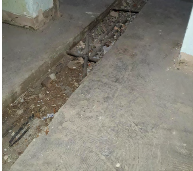
Figure 17 - Ground floor screed over concrete
