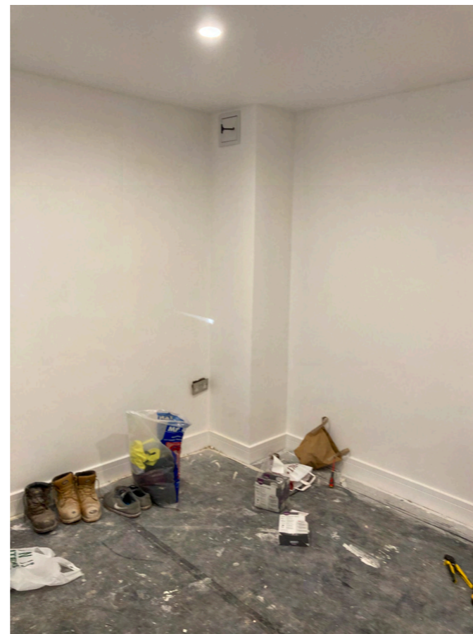
Figure 61 - Boxing out around MVHR ductwork in the corner of a room
