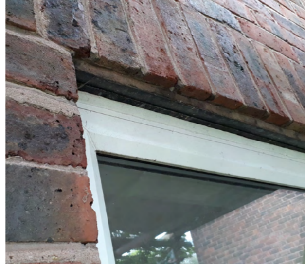
Figure 20 - Metal lintel to window head
