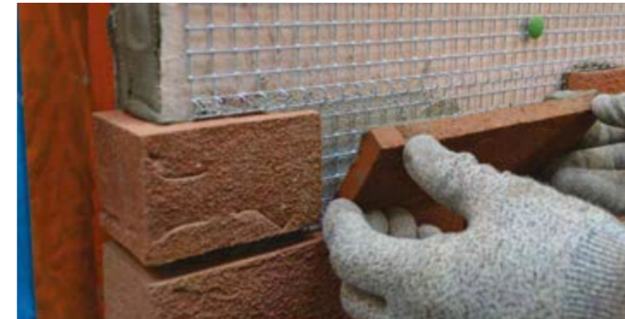
Figure 48 - Brick slips being installed over EWI
