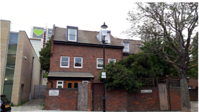
4 Closed off alley by leisure centre
