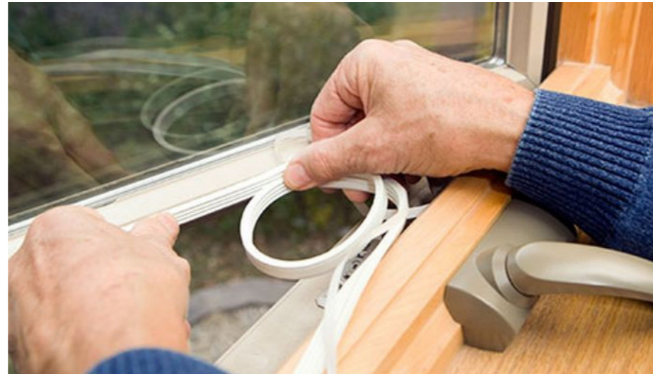
Figure 41 - Installing draught stopping
