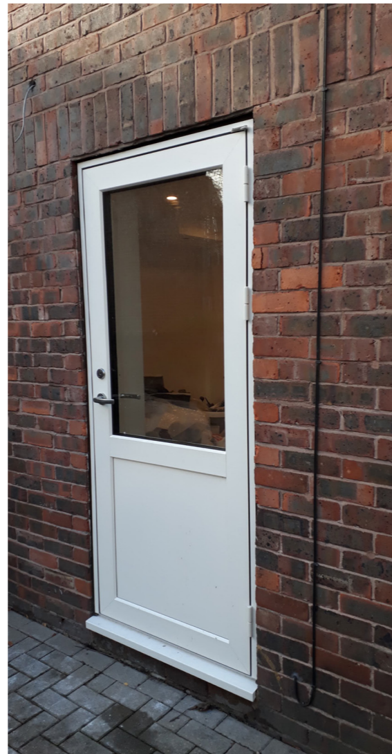
Figure 67 - New insulated triple glazed door at 50 Verity Close
