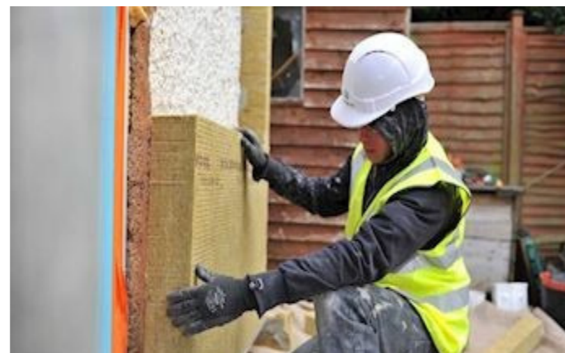
Figure 46 - EWI construction process
