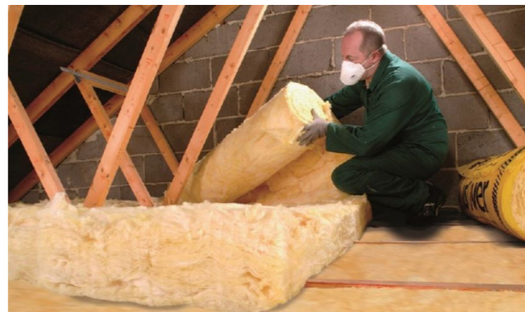
Figure 42 - Installing loft insulation
