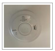
It is imperative that you check that the detector is working weekly by pressing the "test" button on the base of the unit.
