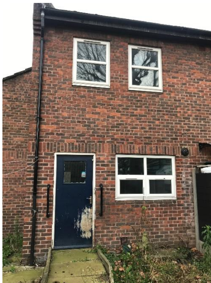
Verity Close preconstruction
