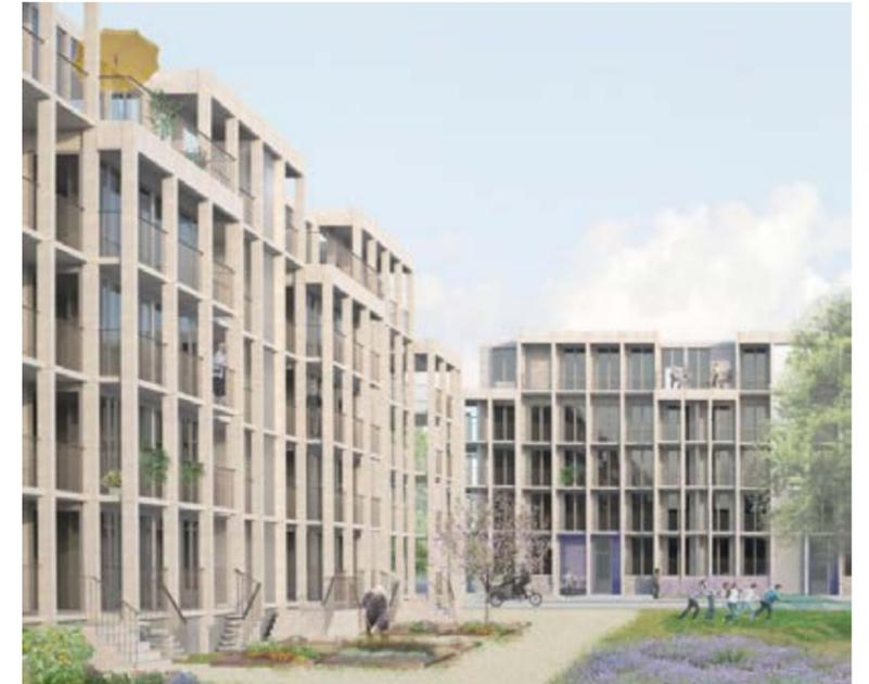
An insulated outer brick skin is being added to the building, with new balconies and stairs down into the communal garden spaces. The skin has completely transformed the appearance of the building, and improved the environmental performance.
