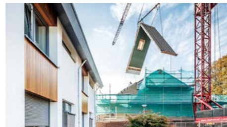
Prefabricated elements to reduce disruption and improve performance
