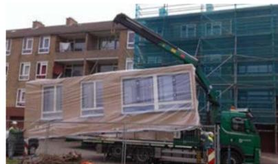
External insulation and prefabricated building elements
