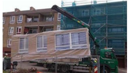
External insulation and prefabricated building elements
