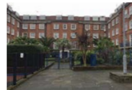
Talbot Grove's courtyard is inaccessible.
