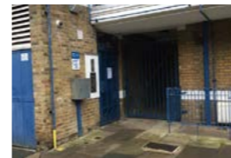
Entrances areas not clearly identified
