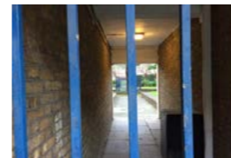
Communal spaces not easily accessible.
