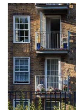
Example of a "bolt-on" balcony
