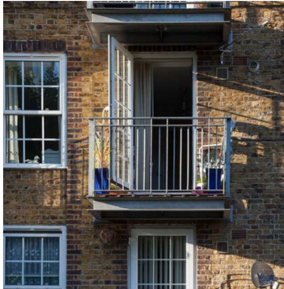
Example of a "bolt on" balcony
