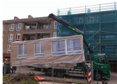
External insulation and prefabricated building elements
