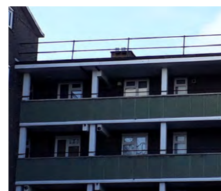
Figure 96 - Existing Roof Railing
