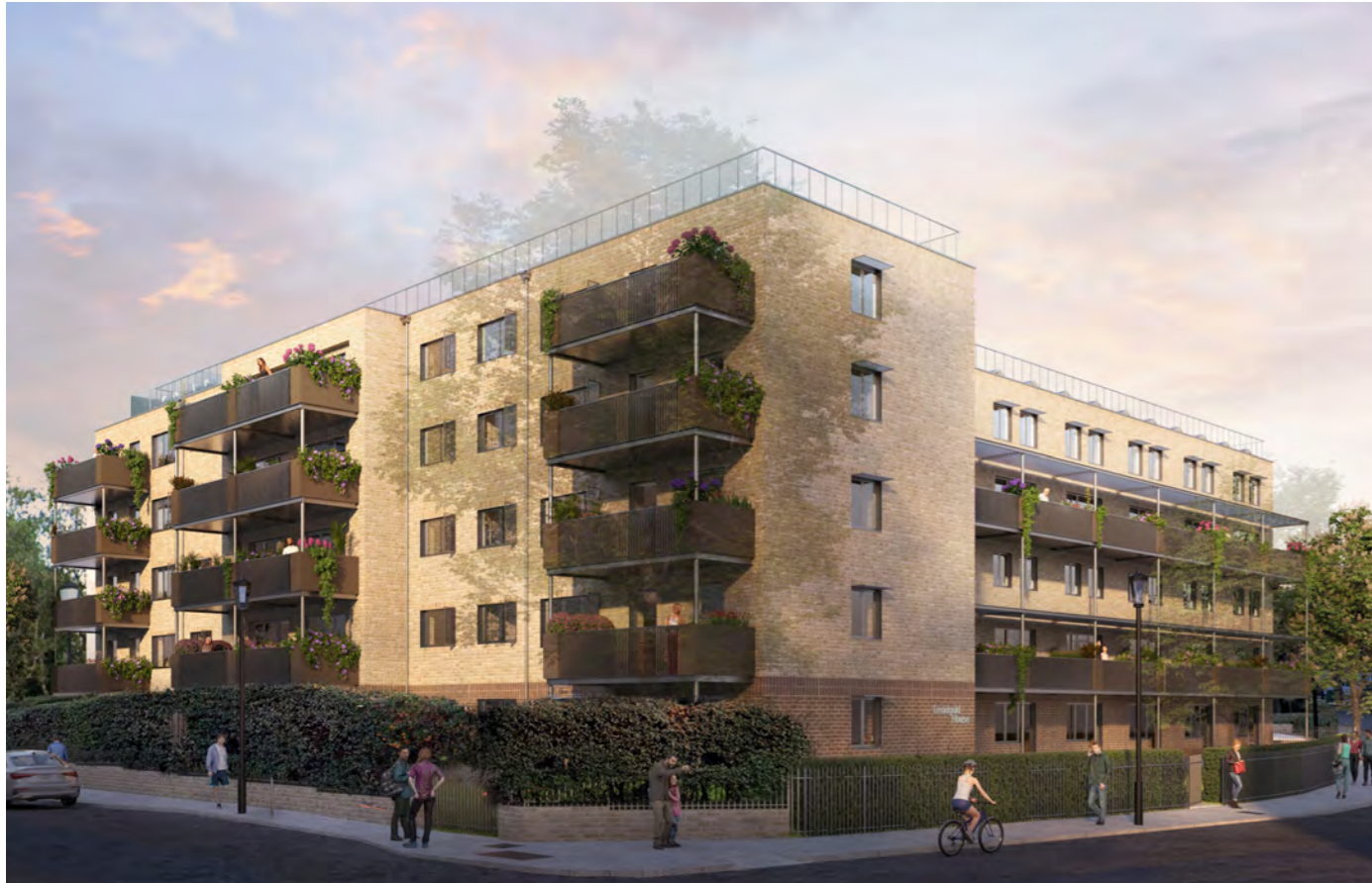
Figure 74 - View of retrofitted Treadgold House from the south west with soldier course brick detailing and darker brick colour highlighting the ground floor
