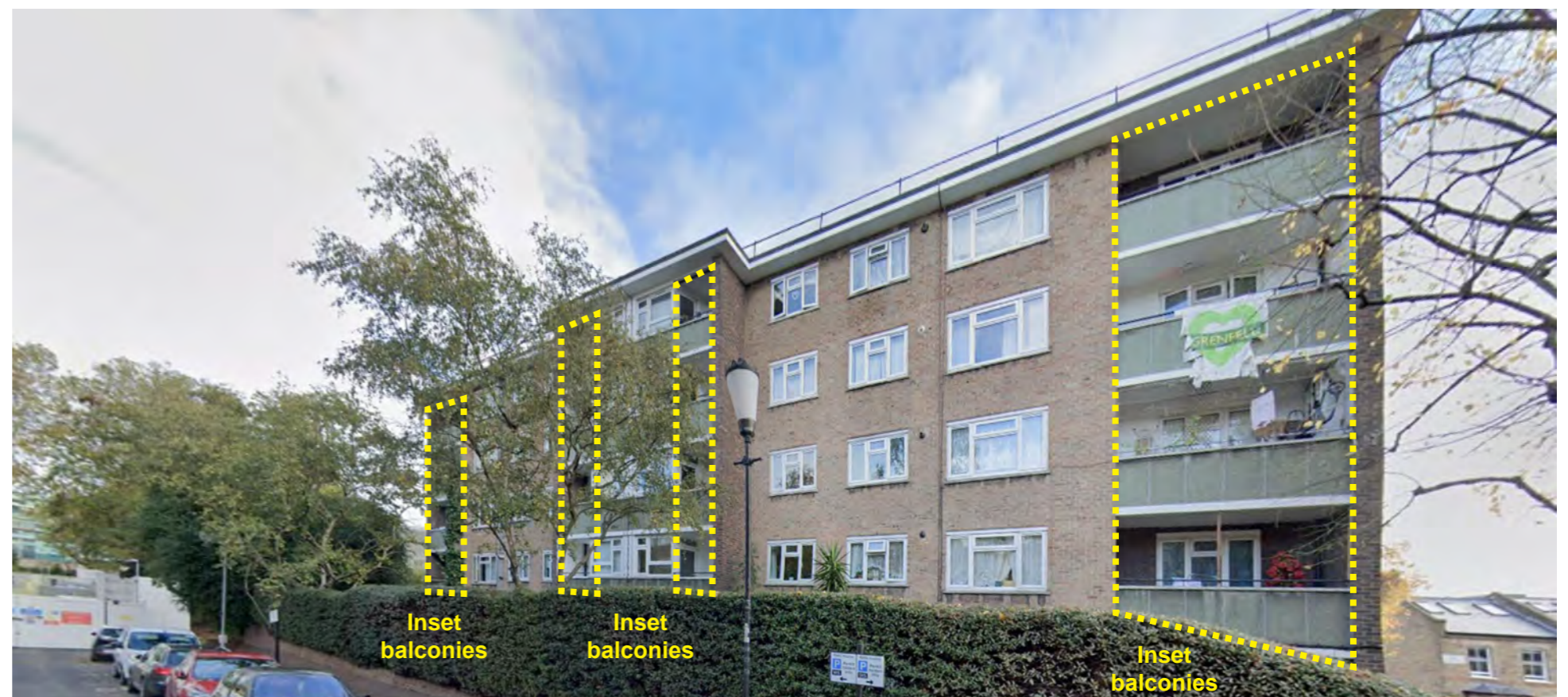
Figure 9 - West wing - West facade
