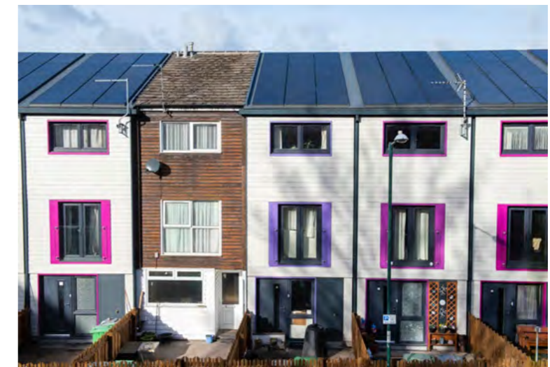
Figure 61 - Melius Homes Modular completed retrofit schemes
