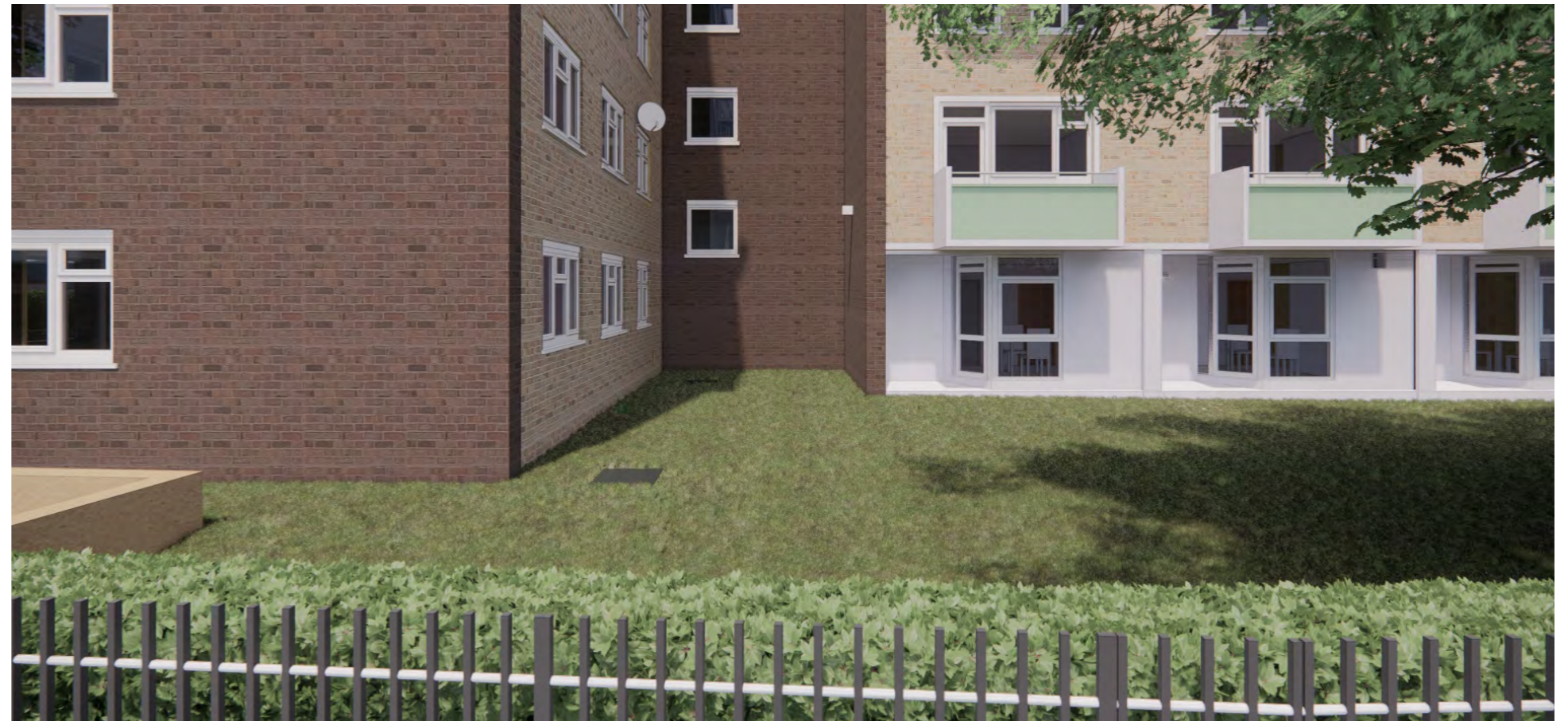
Figure 108 - Existing Front Entrance
