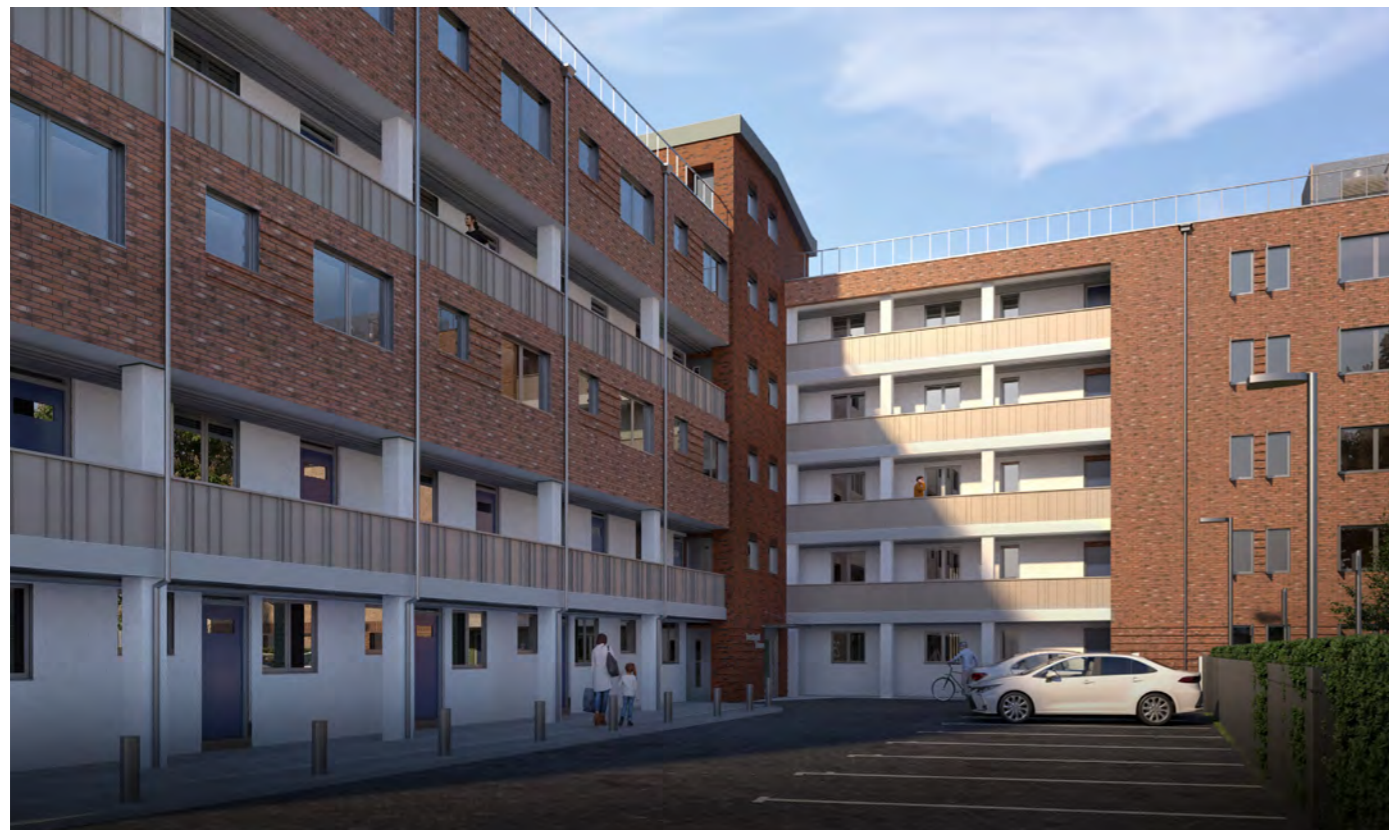
Figure 71 - View of retrofitted Treadgold House from the car park with details of protruding brick composition around the window openings and white render finish in the deck area
