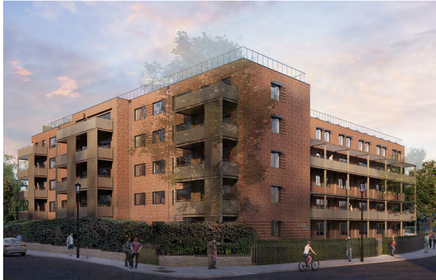
Figure 70 - View of retrofitted Treadgold House from the south west
