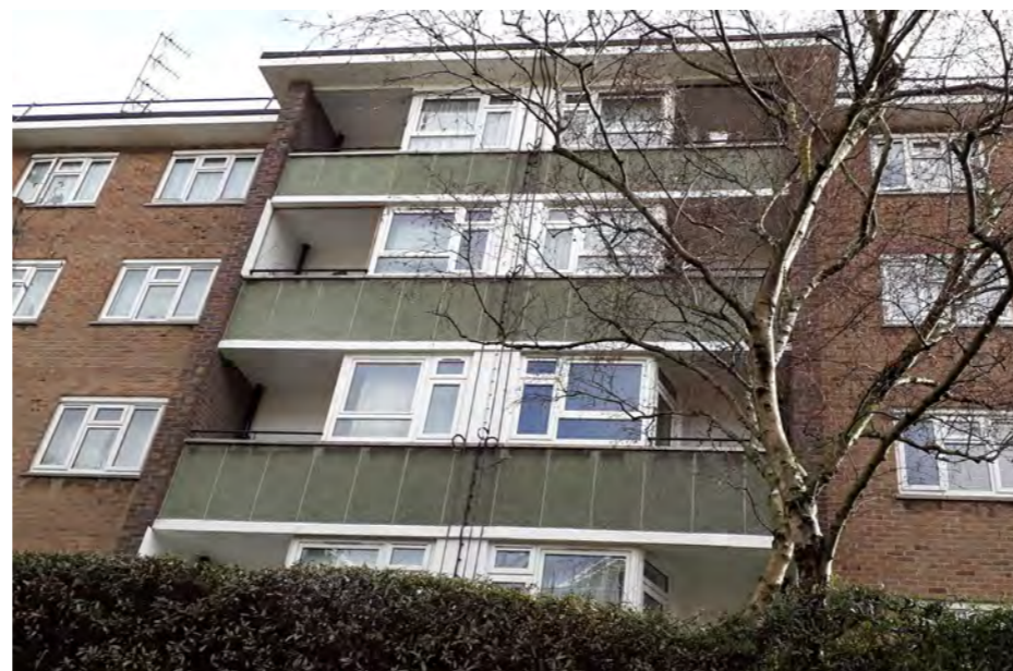
Figure 32 - Rainwater pipes run down rear corner of inset balconies
