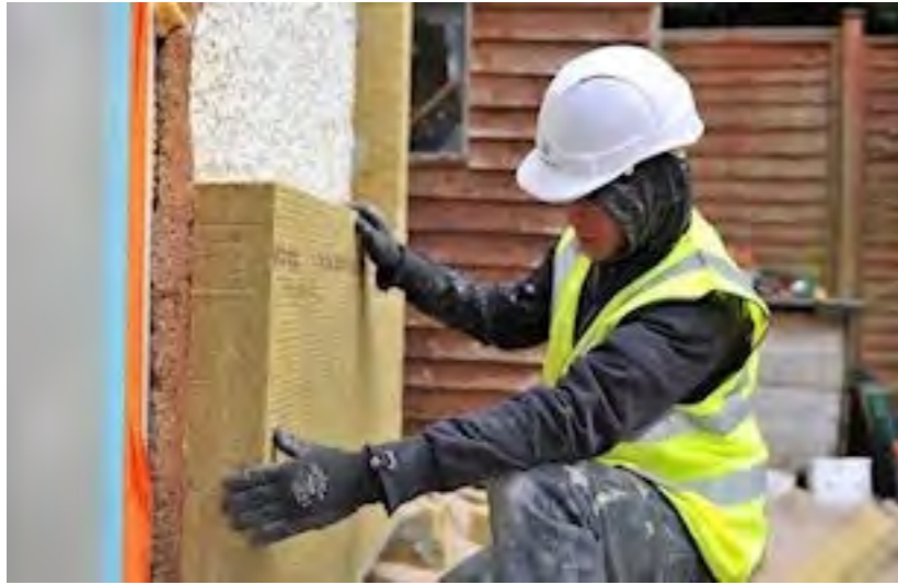
Figure 56 - EWI construction process
