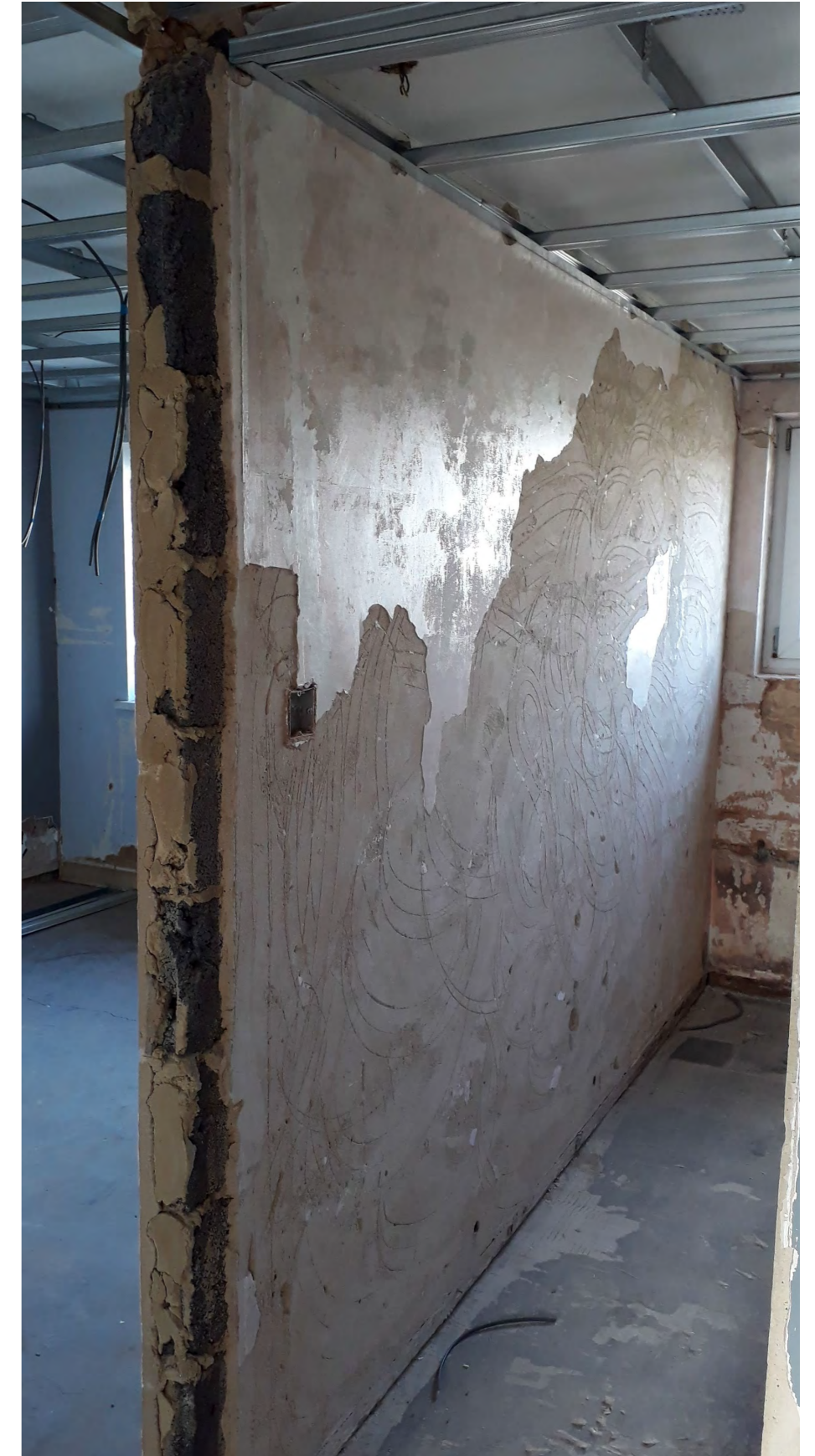
Figure 15 - Block work internal partitions
