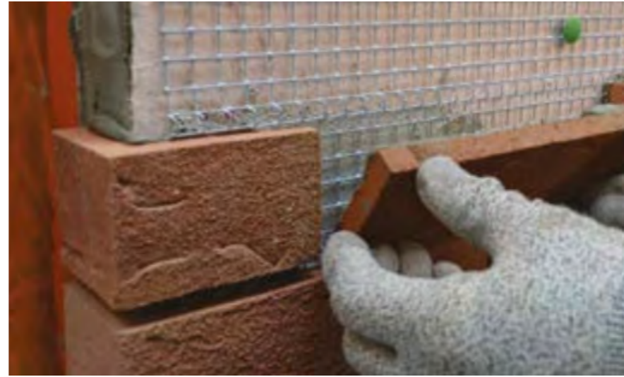
Figure 55 - Brick slips being installed over EWI
