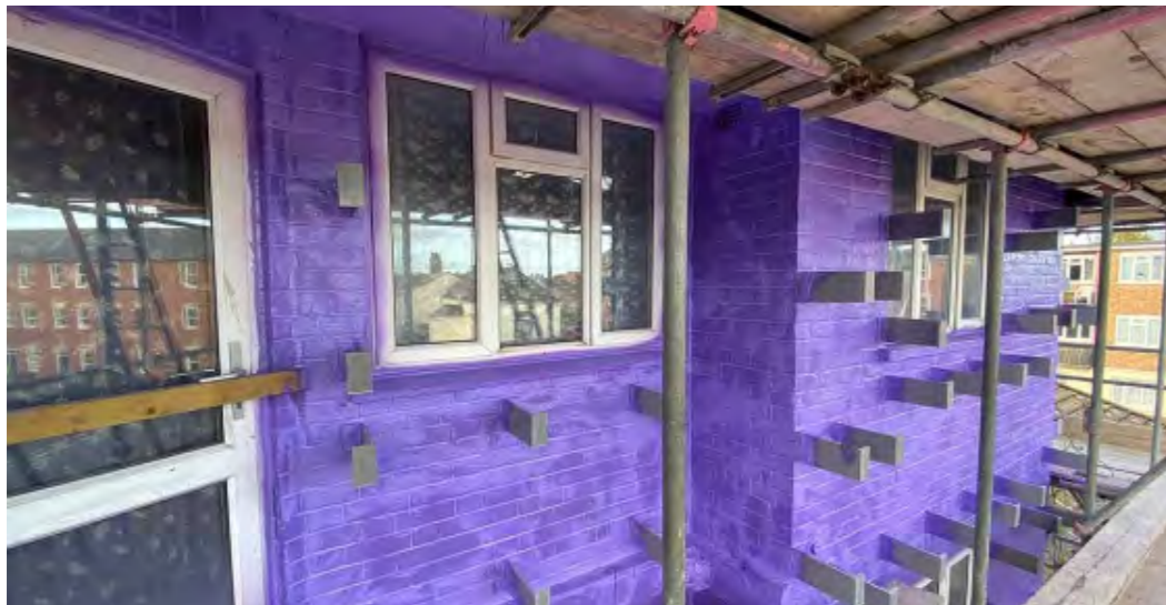
Figure 60 - Beattie Passive system construction process
