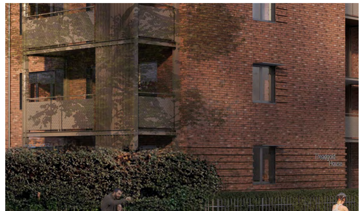
Figure 72 - Detail showing protruding brick detail to pick out ground floor and around windows, as well as vertical shading to west facing balconies
