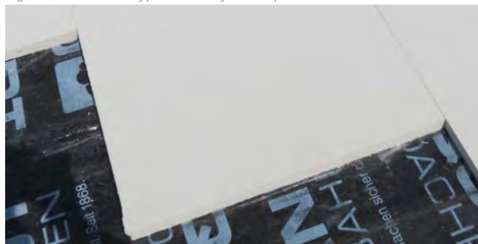
Figure 49 - Calostat boards being installed
