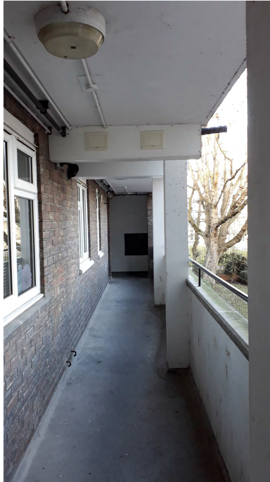
Figure 81 - View down current open access deck
