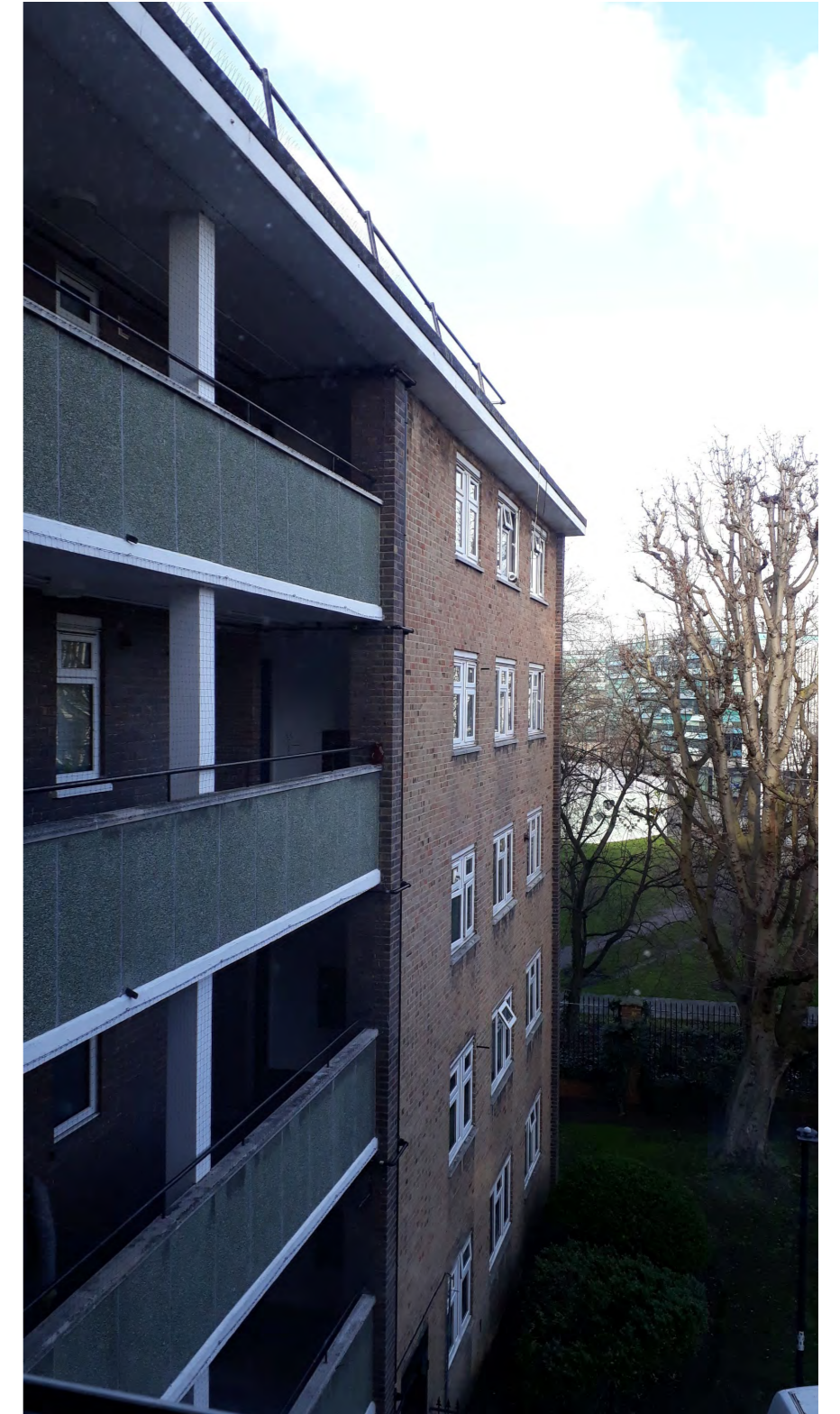
Figure 82 - View of access decks to west wing flats
