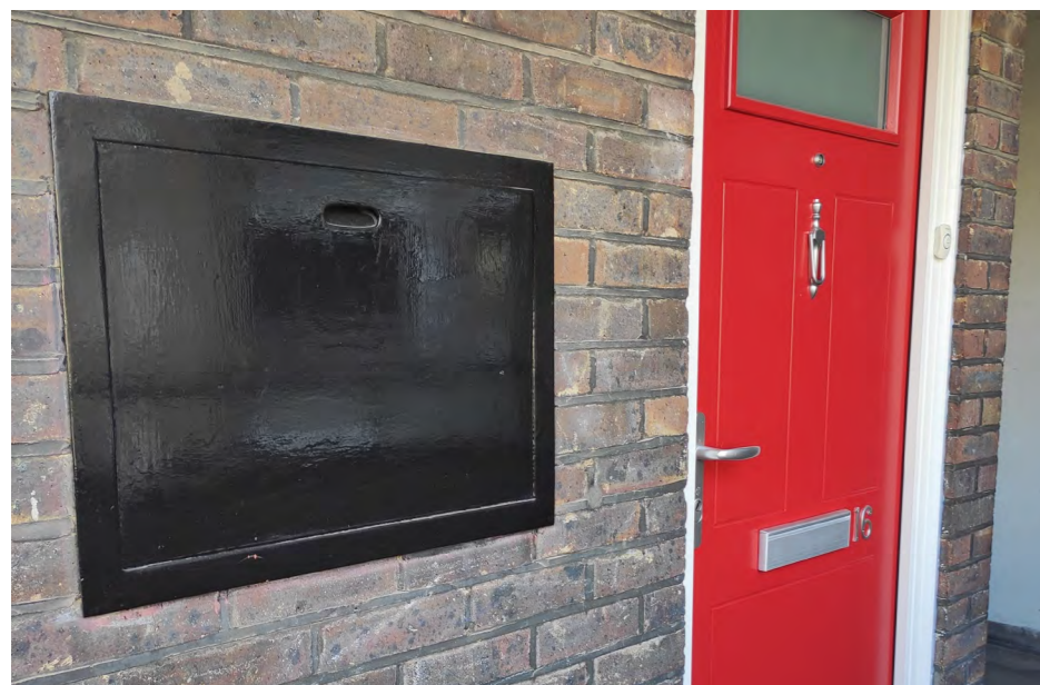
Figure 35 - Coal chute door
