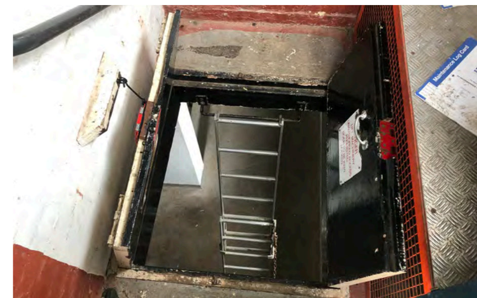
Figure 17 - Access to the roof from above
