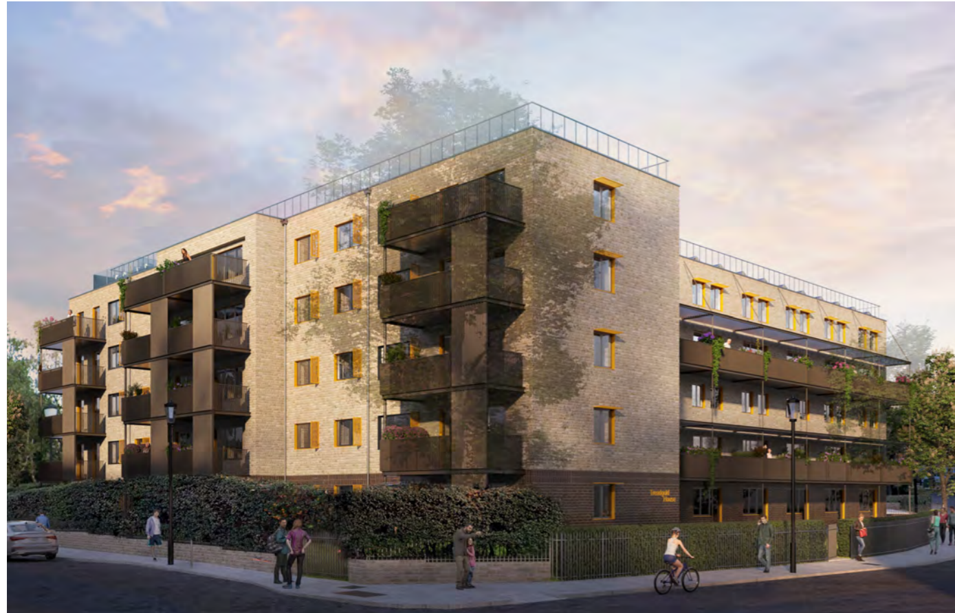
Figure 78 - View of retrofitted Treadgold House from the south west with details of yellow powder coated aluminium frame around the window openings
