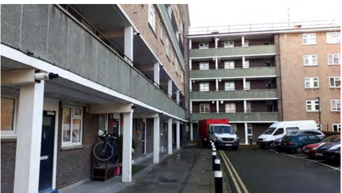
3 Treadgold House car parking
