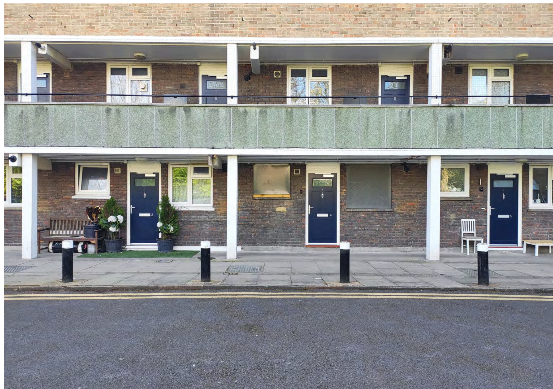
Figure 106 - Existing doors to flats
