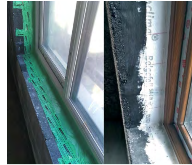
Figure 57 - Airtight window installation
