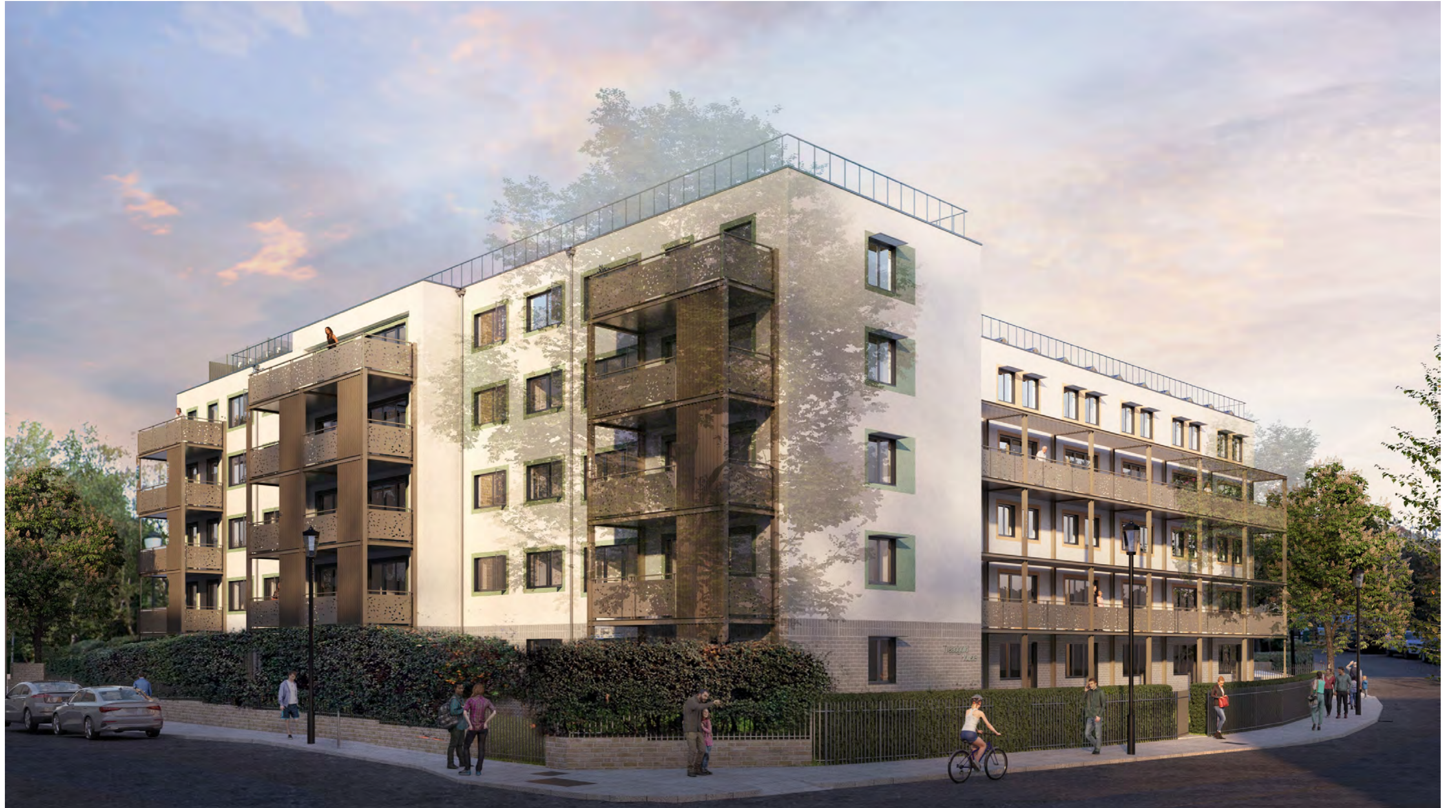
Figure 67 - View of retrofitted Treadgold House from the south west with white render finish and pastel render details around the window openings. The ground floor is a pale grey brick, to add durability where the building meets the ground.
