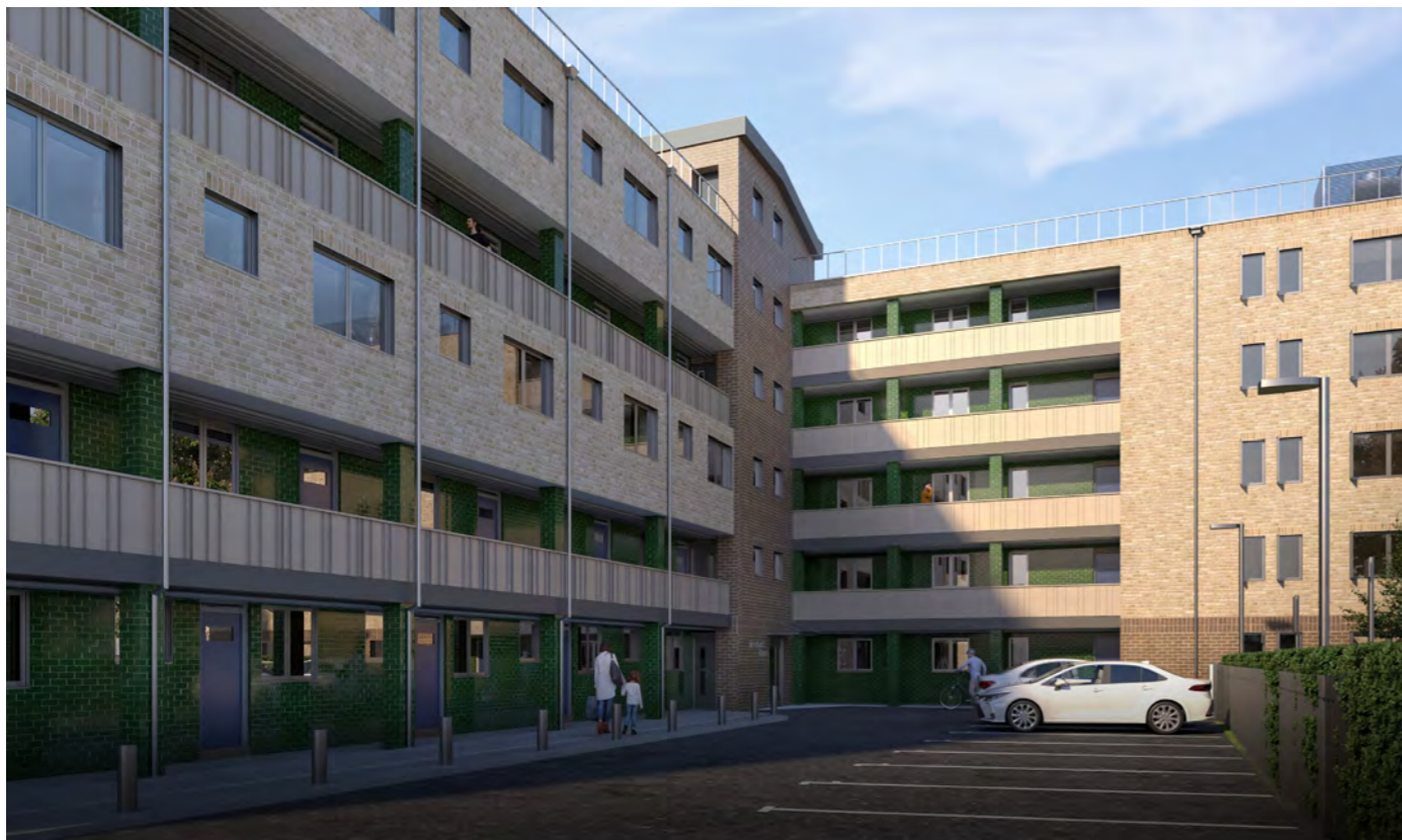
Figure 75 - View of retrofitted Treadgold House from the car park with details of different brick composition along the stairwell to highlight the building's volumes
