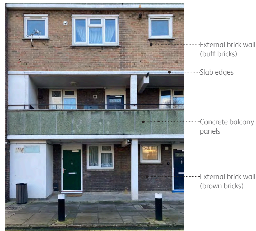
Figure 10 - East wing - North facade
