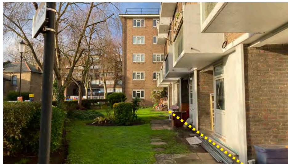
Figure 13 - Assumed Concrete foundation edge line (view from the main gate)
