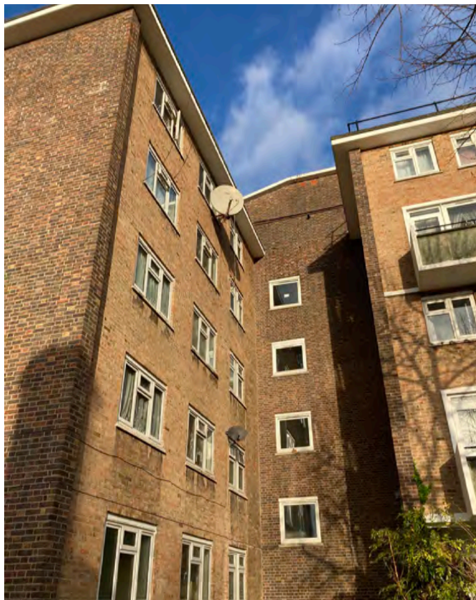
2 Treadgold House staircore from Bomore Road
