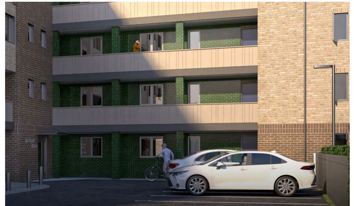
Figure 76 - Detail showing green glazed bricks to walls & columns to deck areas
