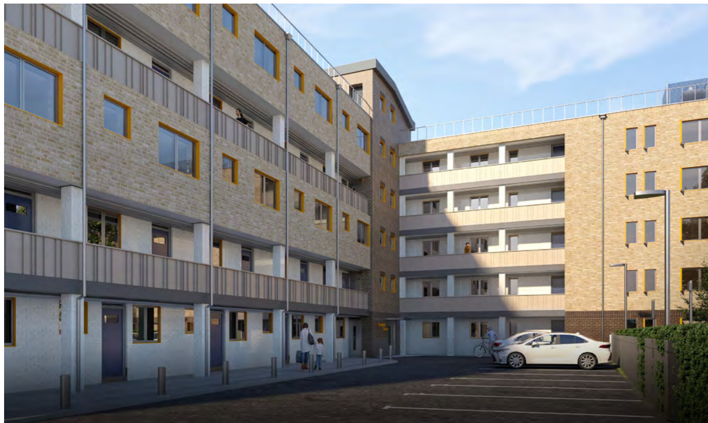
Figure 79 - View of retrofitted Treadgold House from the car park with details of yellow powder coated aluminium frame around the window openings and white glazed bricks to deck areas.
