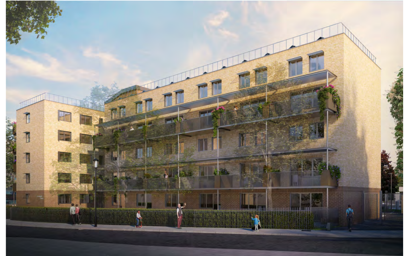
Figure 73 - View of retrofitted Treadgold House from the south east with soldier course brick detailing and darker brick to ground floor
