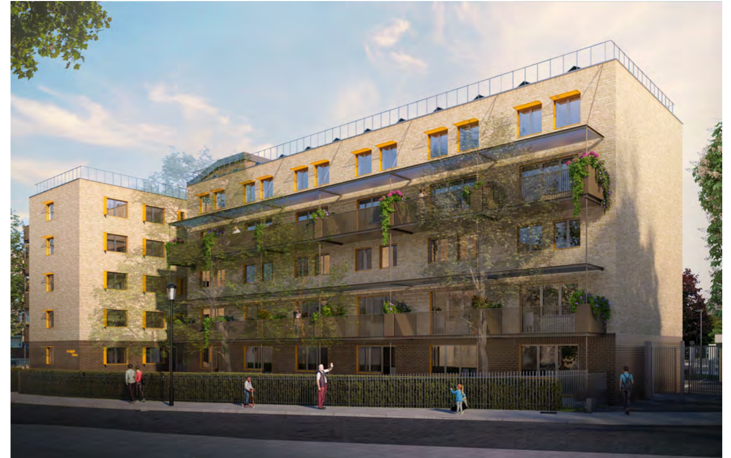
Figure 77 - View of retrofitted Treadgold House from the south east, showing balcony structure partially supported from above
