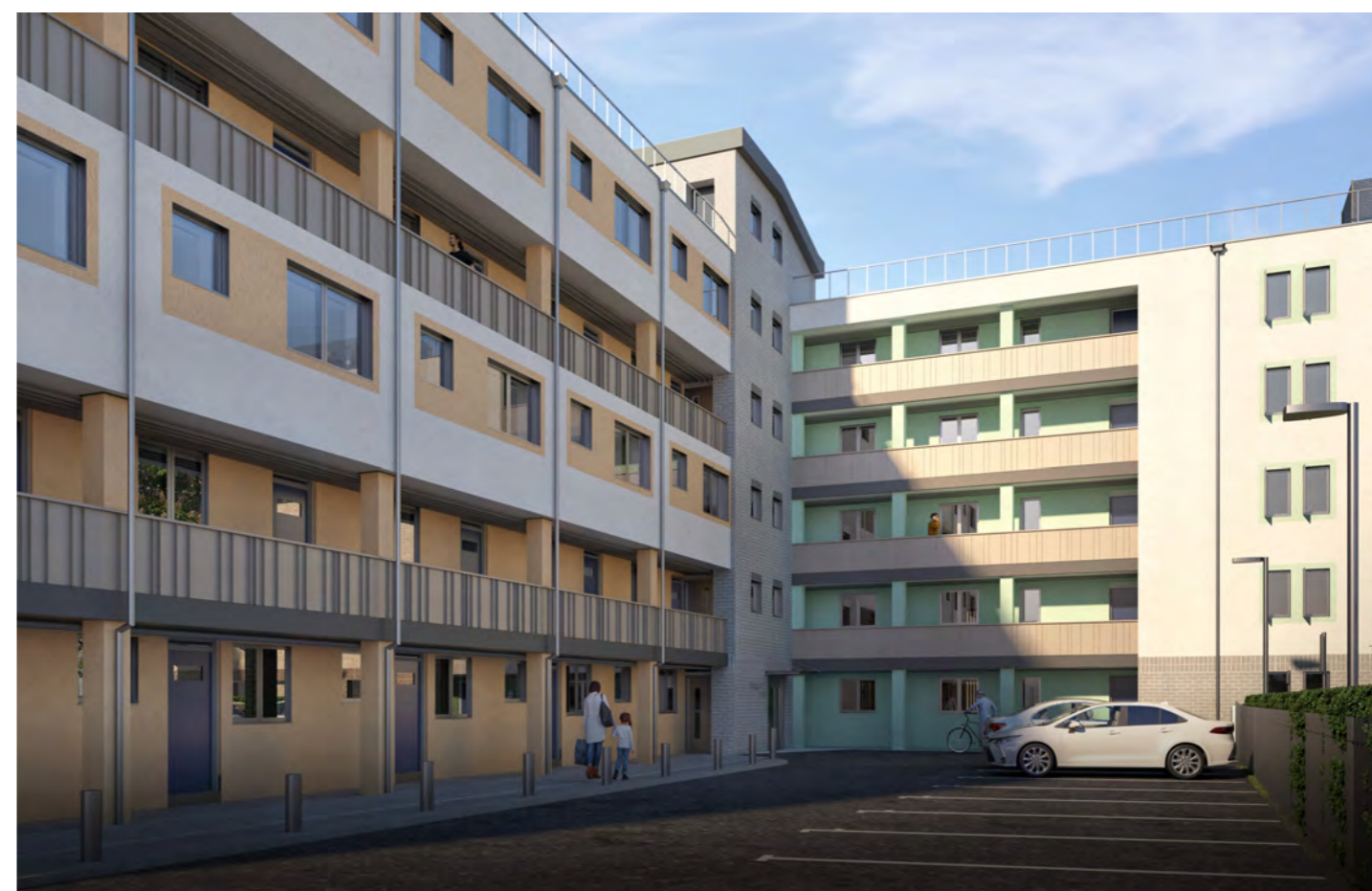
Figure 66 - View of retrofitted Treadgold House from the car park with white render finish and pastel render details to pick out the deck areas
