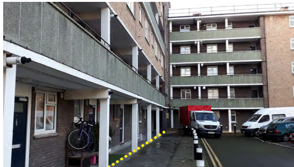
Figure 12 - Assumed Concrete foundation edge line (view from the car park)
