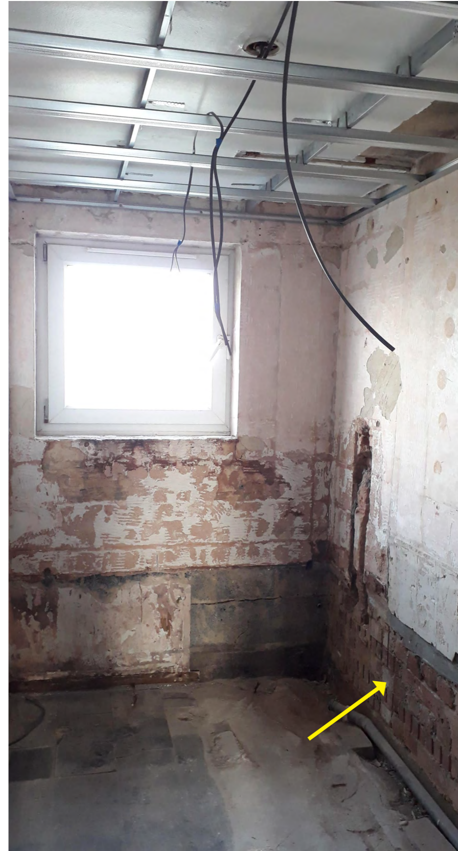
Figure 14 - Brick separating walls
