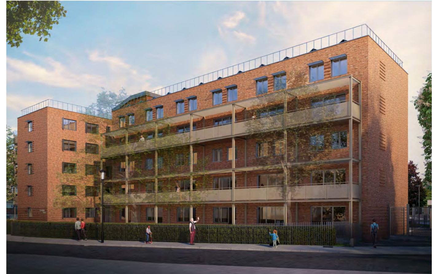
Figure 69 - View of retrofitted Treadgold House from the south east, with perforated balcony balustrade and protruding brick detailing between windows and to the east wall
