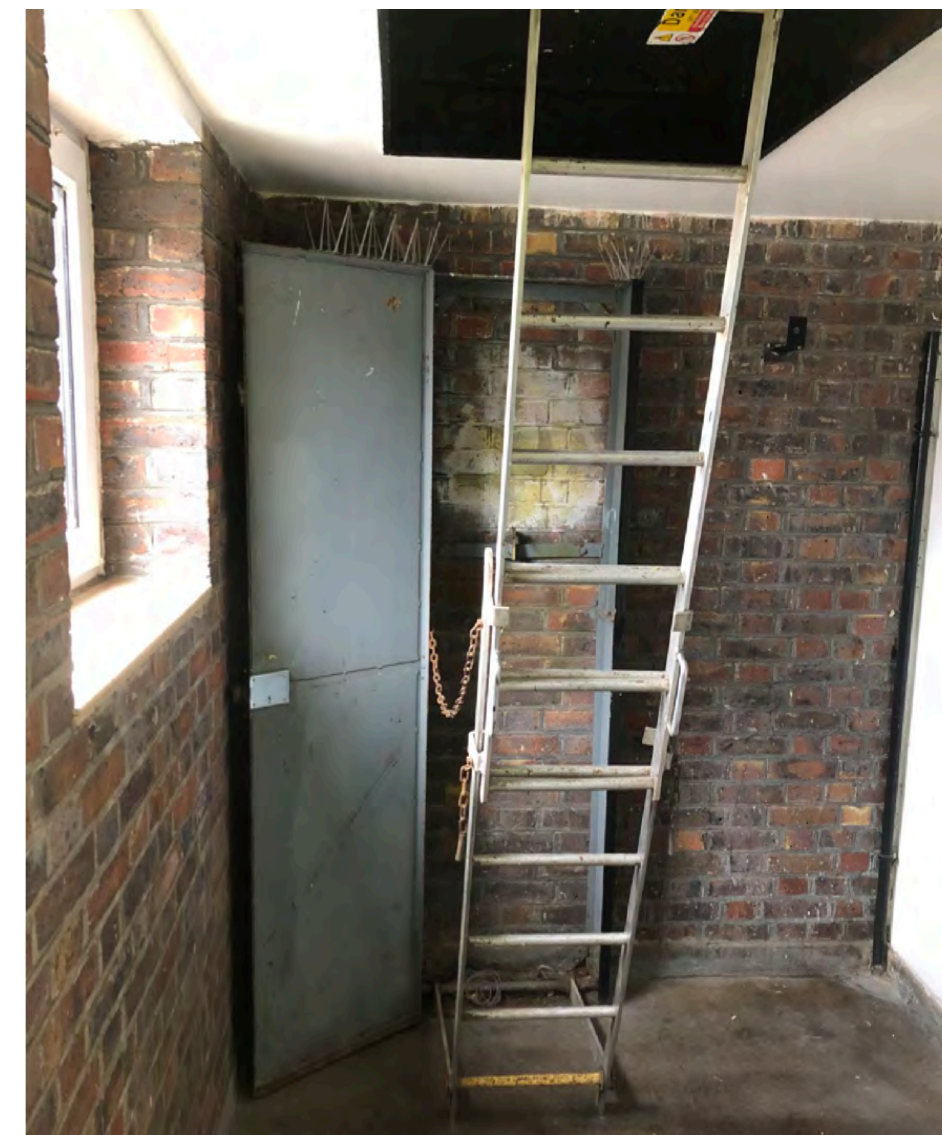
Figure 16 - Access to the roof from the third floor
