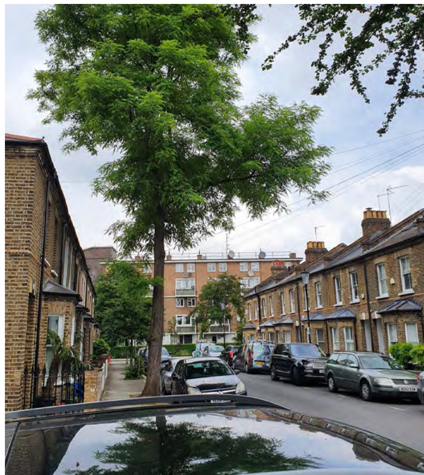
Figure 130 - Treadgold House seen from Treadgold Street
