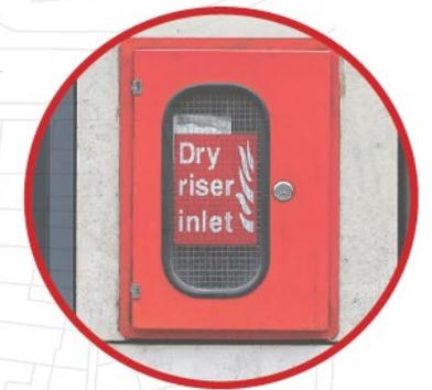
New Dry Riser Inlets: Can be installed in strategic locations to help with fire servicing.
