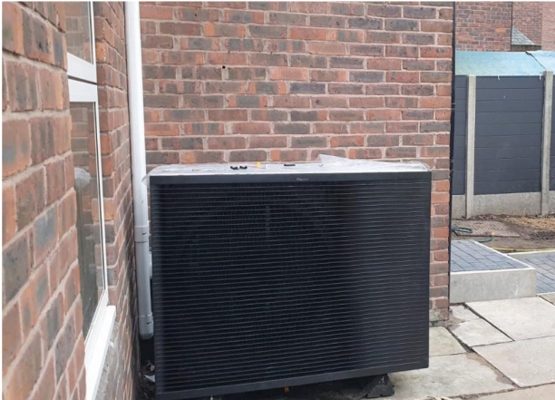
Figure 22 - Air source heat pump external unit
