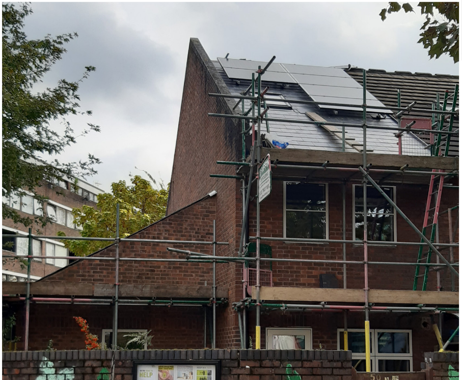
Figure 12 - The home as roof works were completed
