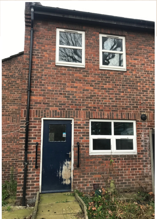
Figure 7 - The home at Verity Close prior to retrofit
