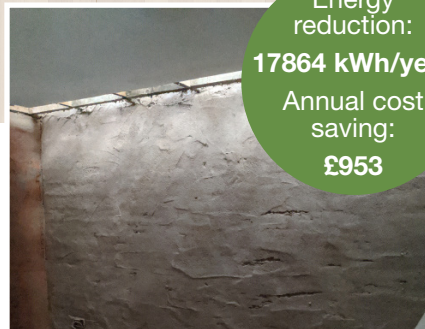
Figure 14 - Walls with internal insulation freshly applied
