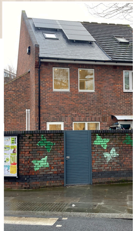
Figure 25 - ...and to the west side of the roof
