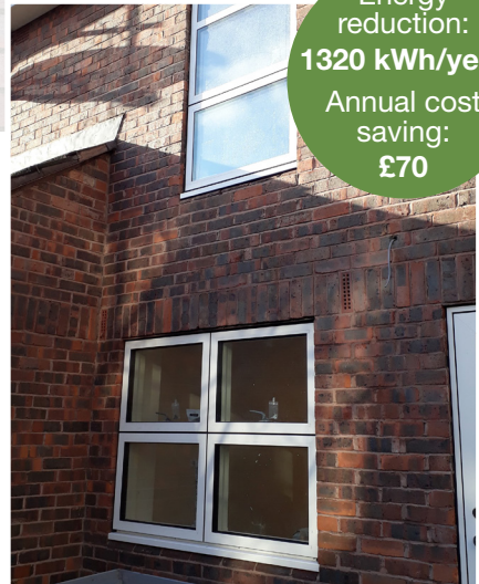
Figure 18 - Window frames are airtight and better insulated but still appear relatively 'light' externally
