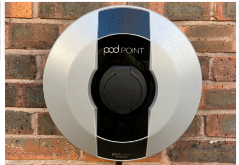
Figure 28 - Electric car charging point
