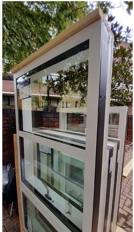
Figure 16 - New windows being delivered to site
