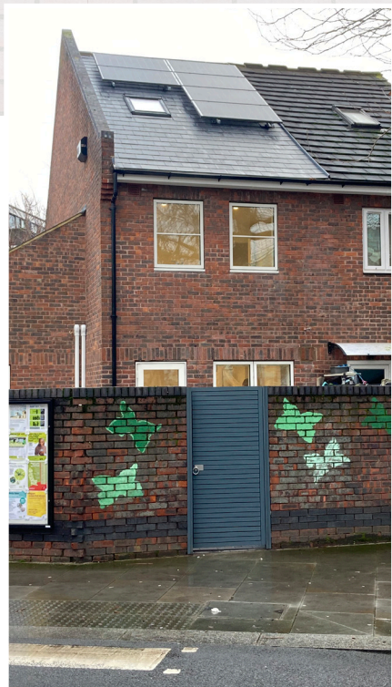
Figure 2 - Post-retrofit, with new windows & photovoltaic panels
