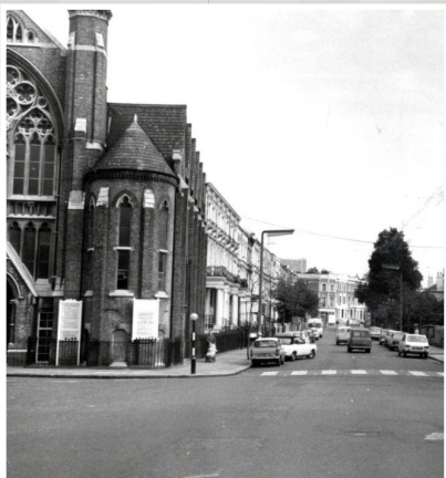
Figure 4 - Notting Hill Methodist Church, pictured in the 1960s
