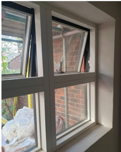
Figure 17 - New windows, designed to open similarly to existing windows
