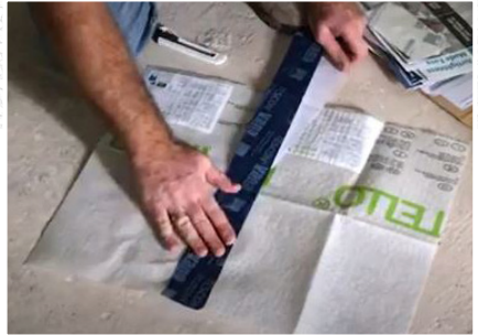
Figure 29 - Practicing airtightness taping on a small scale
