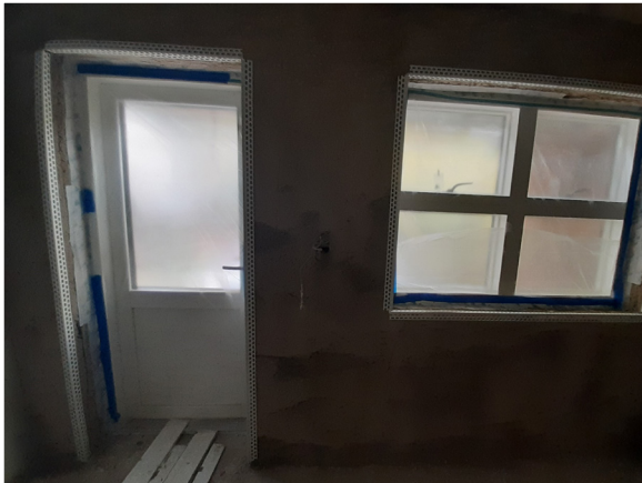
Figure 30 - Window & door installed with airtightness tape sealing them to the walls
