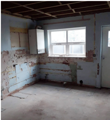
Figure 6 - Kitchen before works
