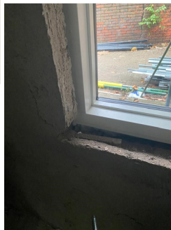
Figure 34 - Insulation creates a thicker wall
